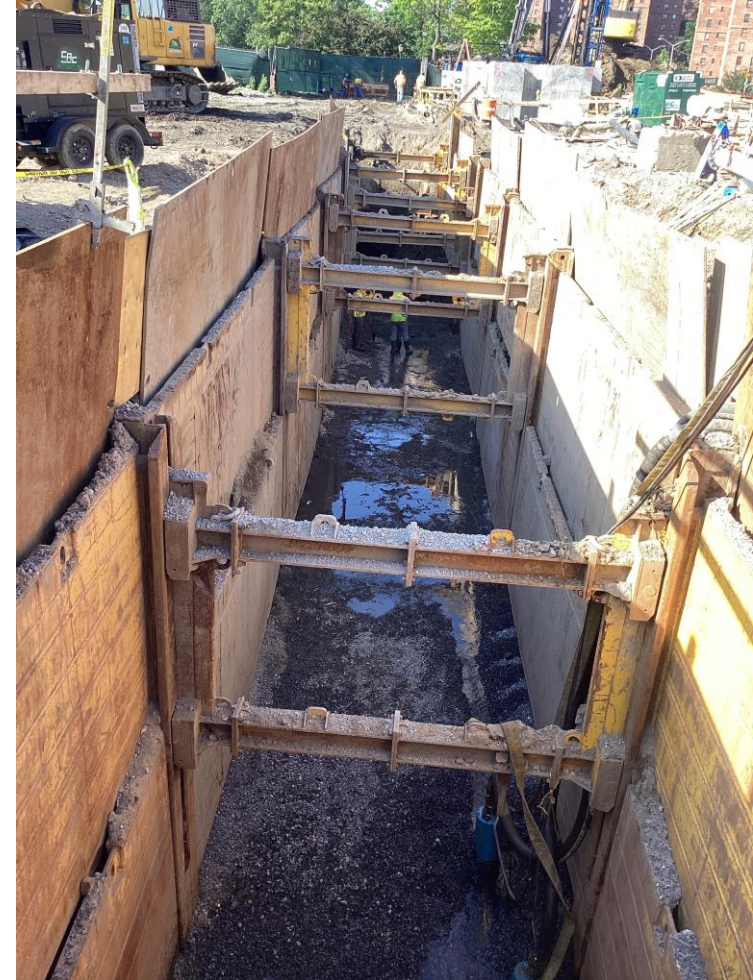
Deep sewer trench north of Track – June 2025
