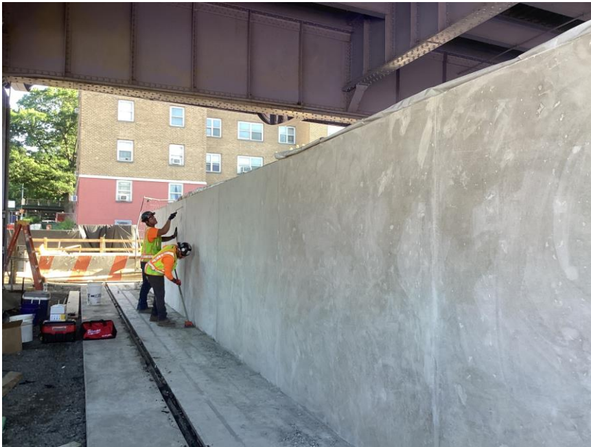
Floodwall at location of future floodgate – June 2025
