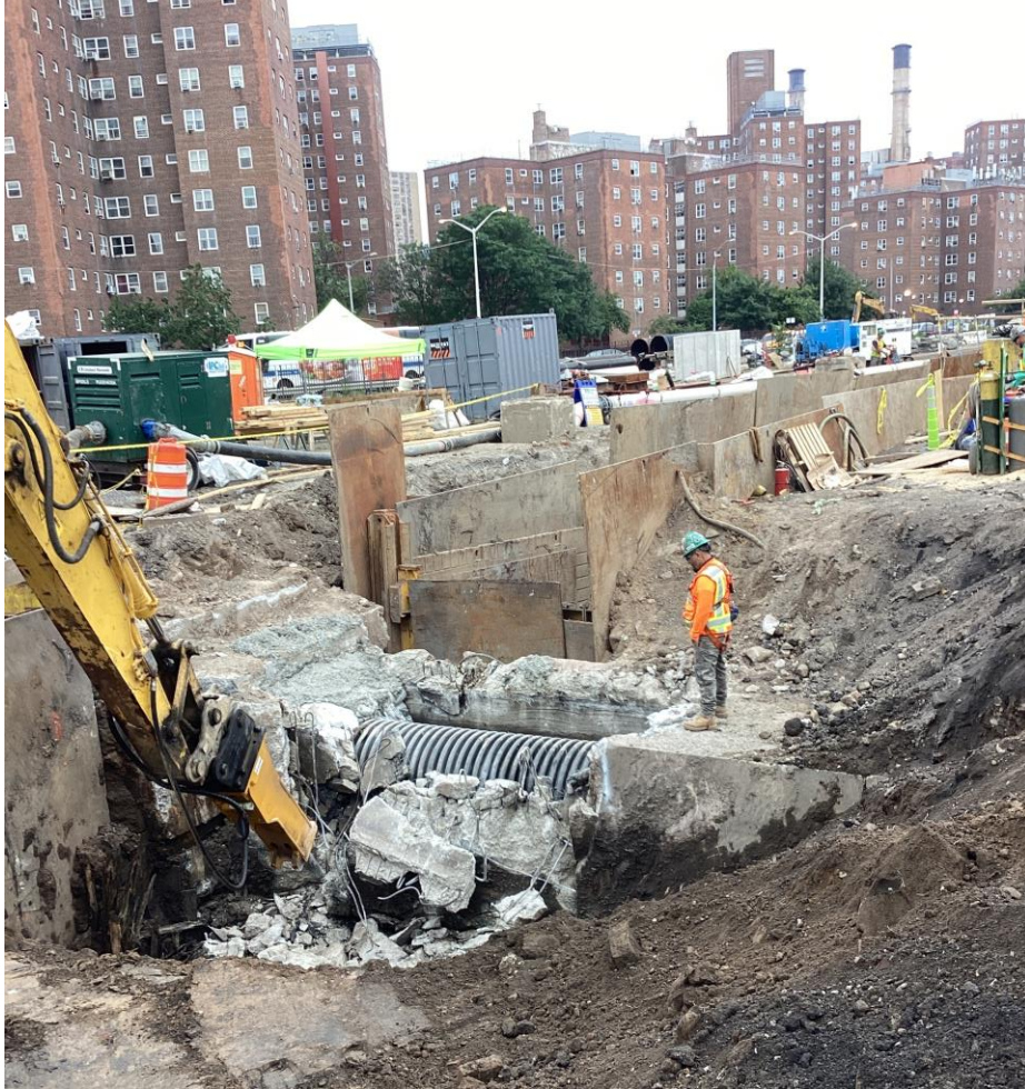
Excavating for deep sewer work north of Track – June 2025
