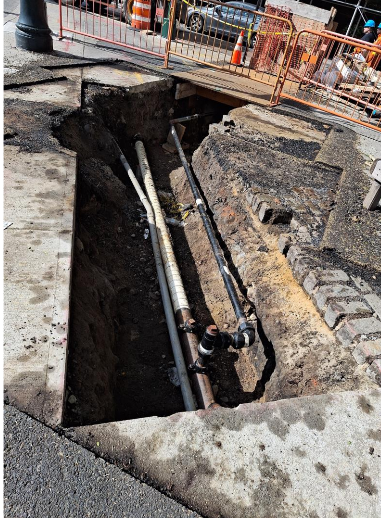
Gas main installation on E. 18 th Street – June 2025
