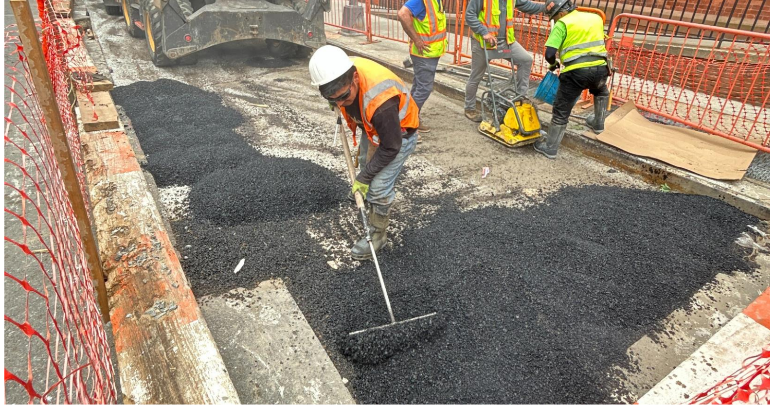
Temporary asphalt installation during South St. restoration – May 2025
