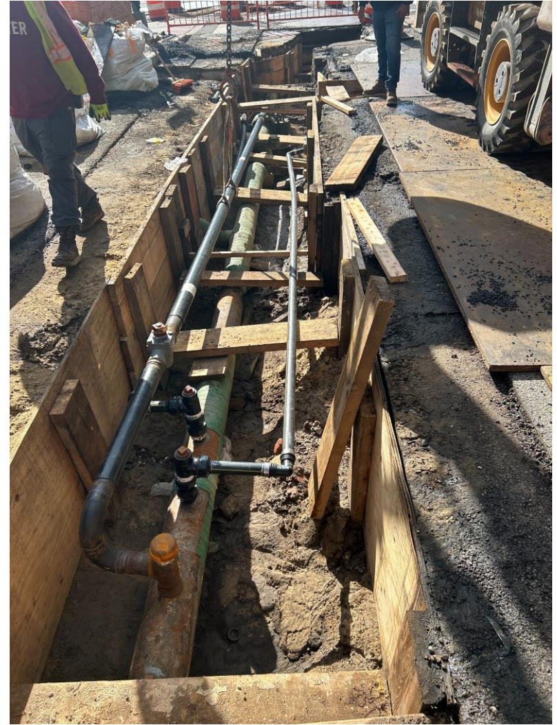
Gas main relocation on E. 18 th St. – May 2025
