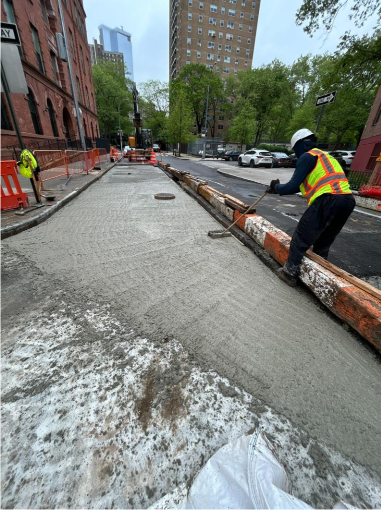
Concrete base for Gouv. Slip E restoration – May 2025
