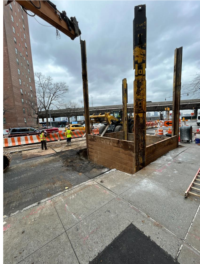
Test pit to locate interceptor sewer in E. 20th St. – March 2025
