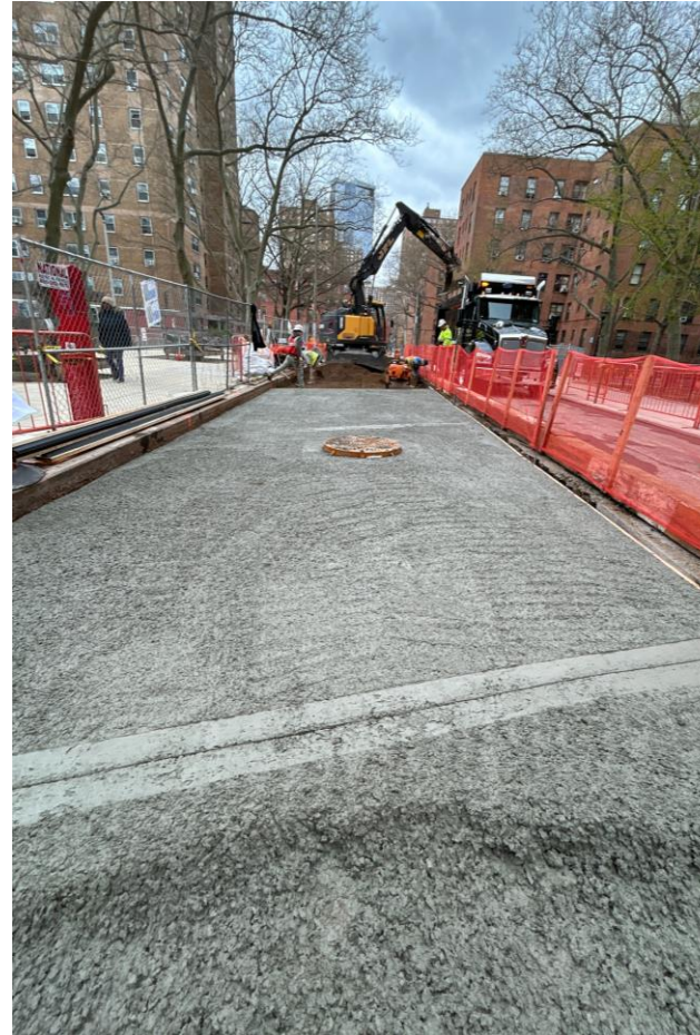
Concrete base for Water St. road restoration – April 2025
