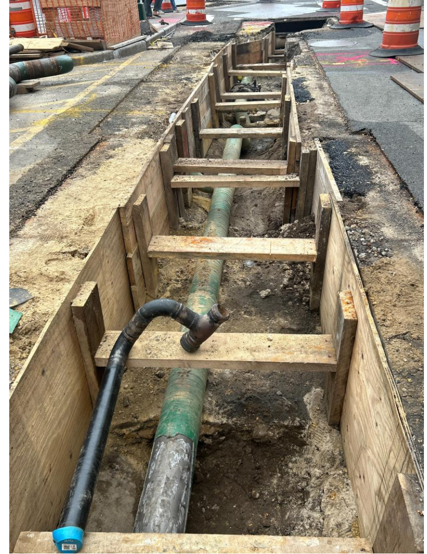
Gas main relocation in E. 18 th St. – April 2025
