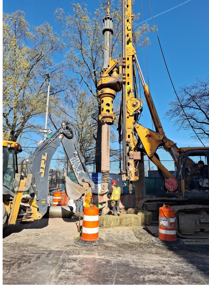
Well point drilling in Jackson St. – April 2025
