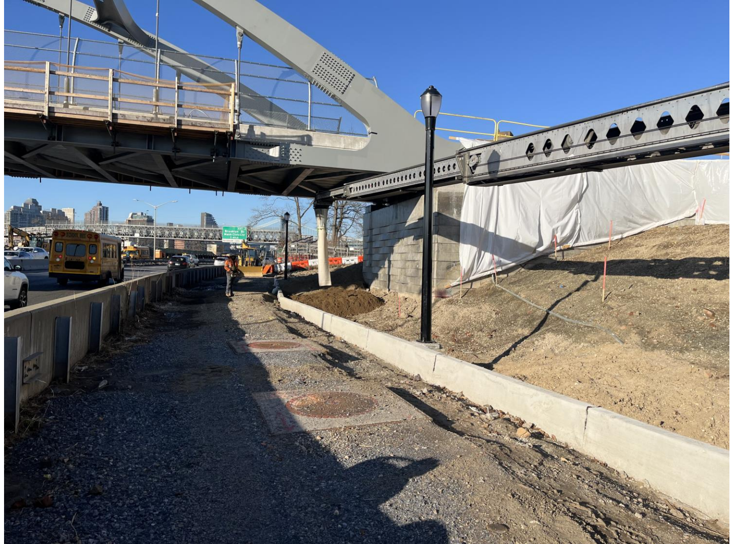
Lighting fixtures and horticultural subsoil installed in Corlears Hook Park – March 2025
