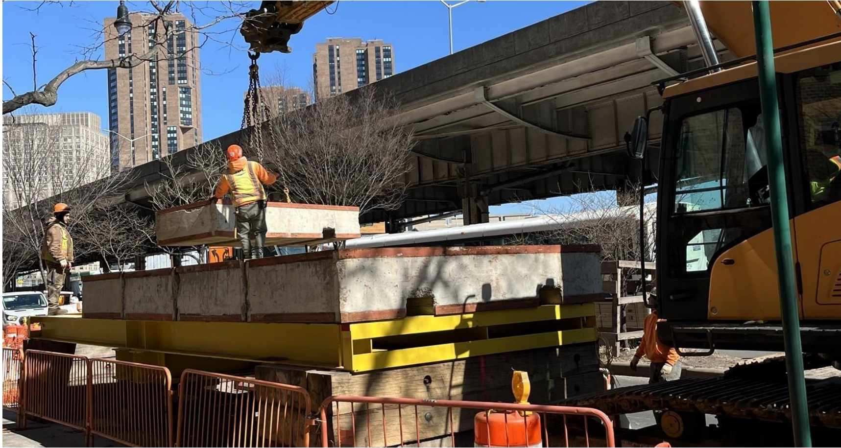
Micropile load test on Avenue C – March 2025
