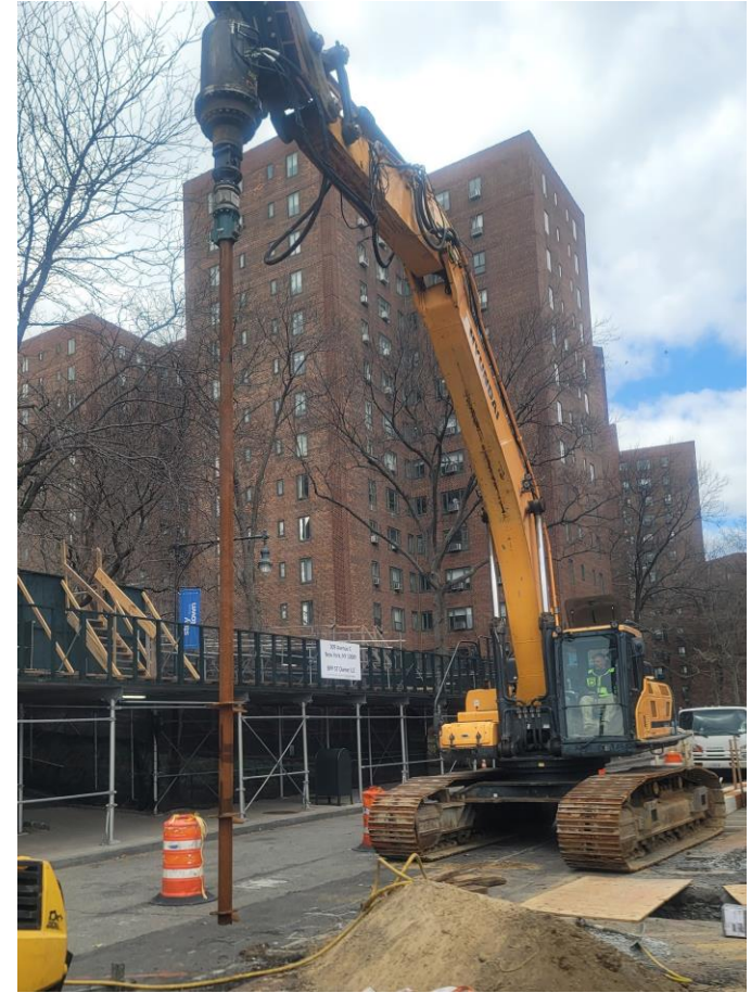
Helical test pile installation in E. 18 th St. – March 2025
