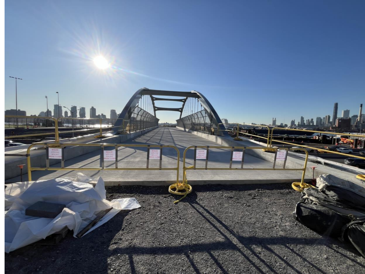
Concrete sealant applied to Corlears Hook Bridge span – March 2025
