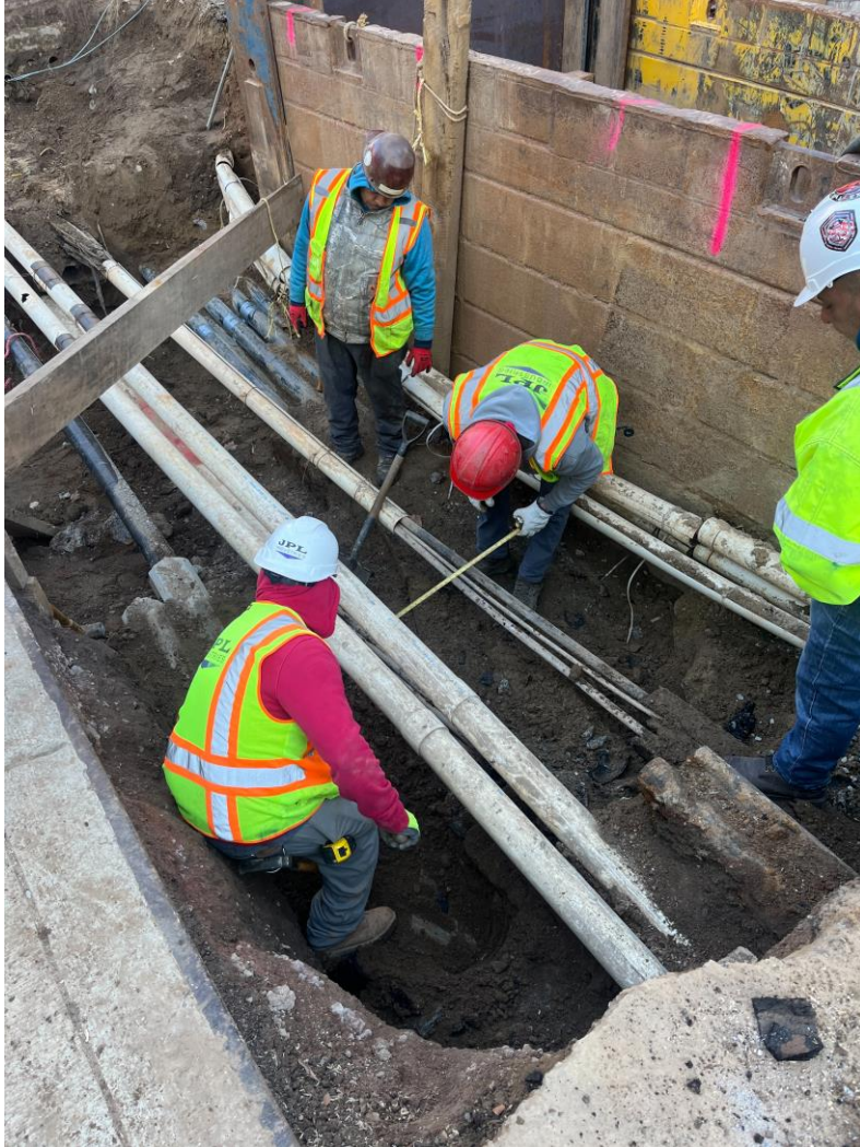
Utility wingback in Water Street - March 2025
