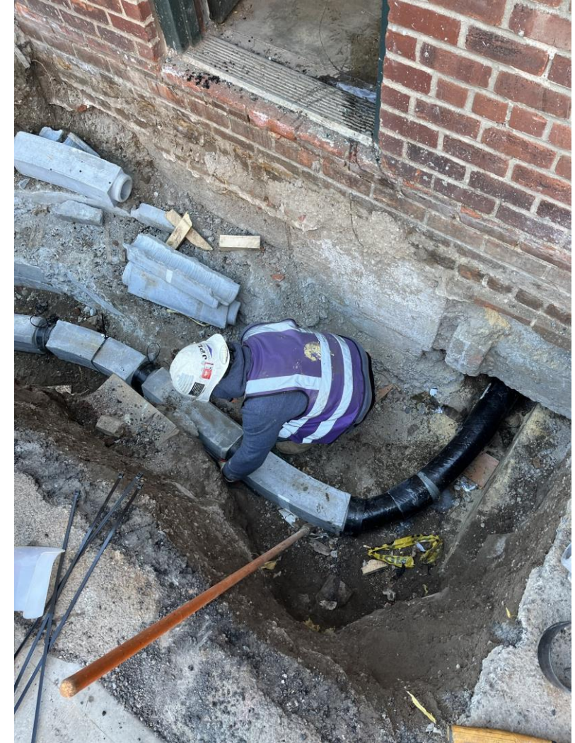
Building service on E. 20 th St. - March 2025
