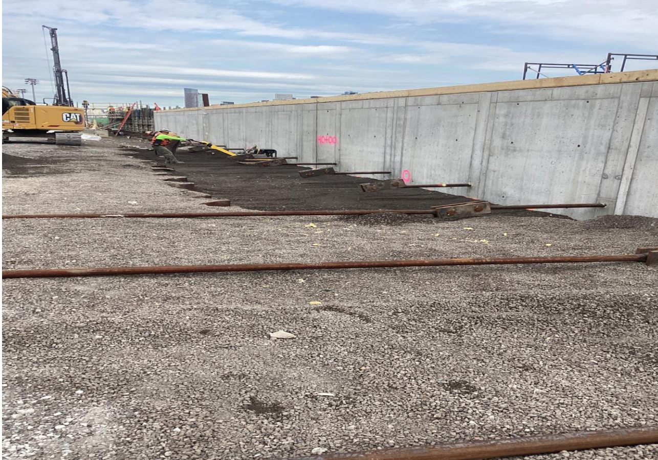
Lightweight fill material installed near tie rods and combi-wall – March 2025
