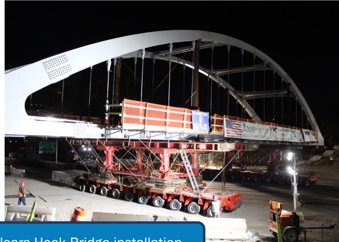
Corlears Hook Bridge installation
