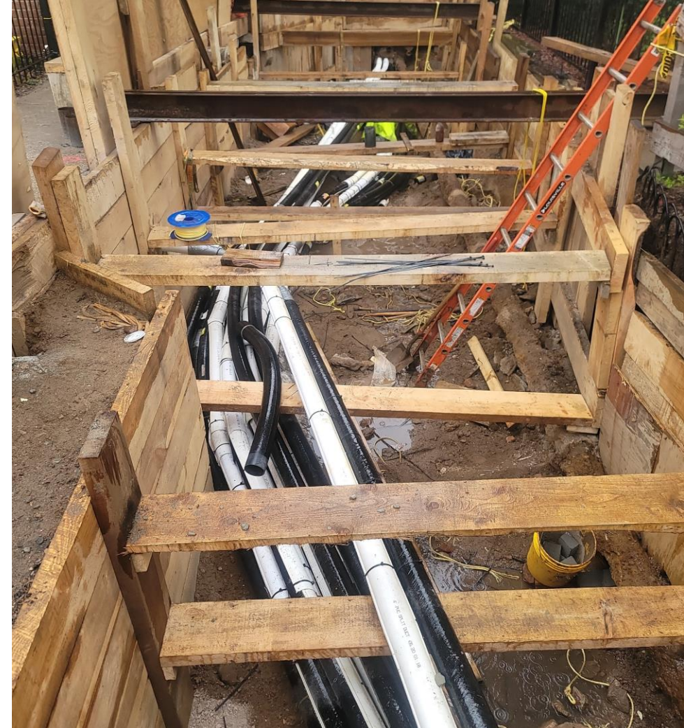
Electric utility relocation in Lewis St. and Broome St. – April 2024
