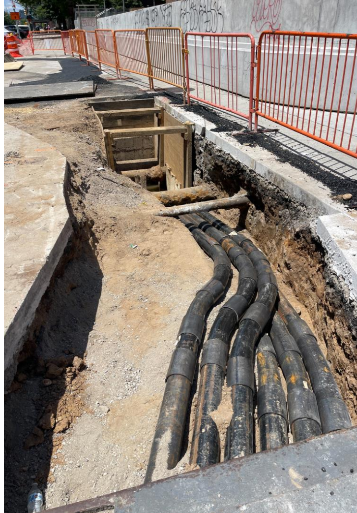
Con Ed duct installation at Delancey St. N and Baruch Drive – May 2024
