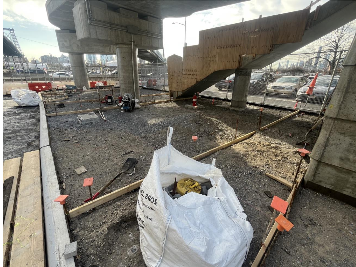
Grading for sidewalk under Delancey Street Pedestrian Bridge – February 2025
