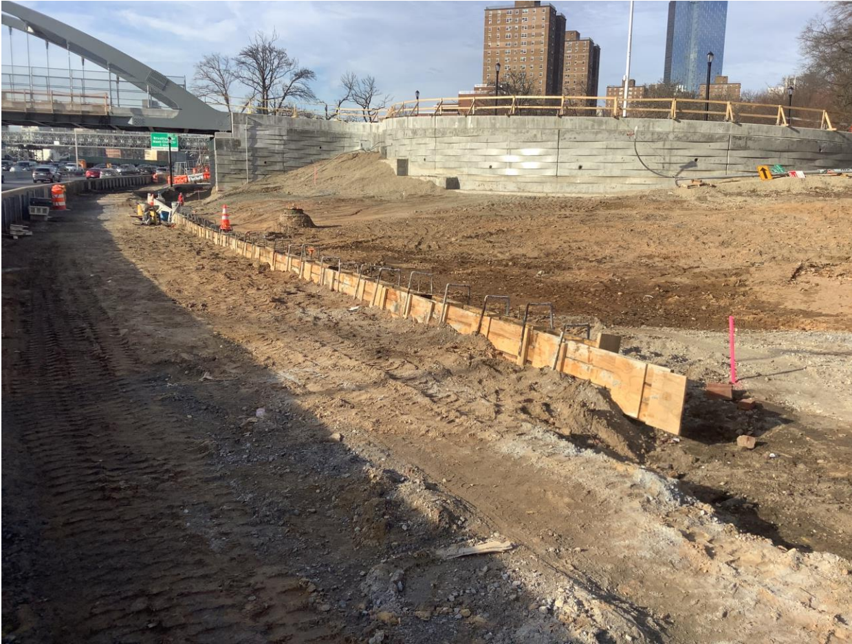
Curb formwork near Corlears Hook bridge – February 2025
