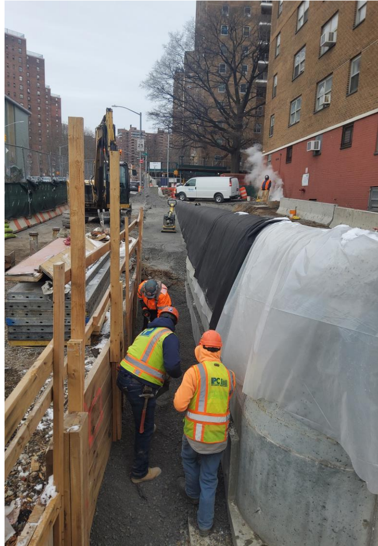
Backfilling floodwall at Montgomery Street and South Street (near Gouverneur Gardens) – January 2025
