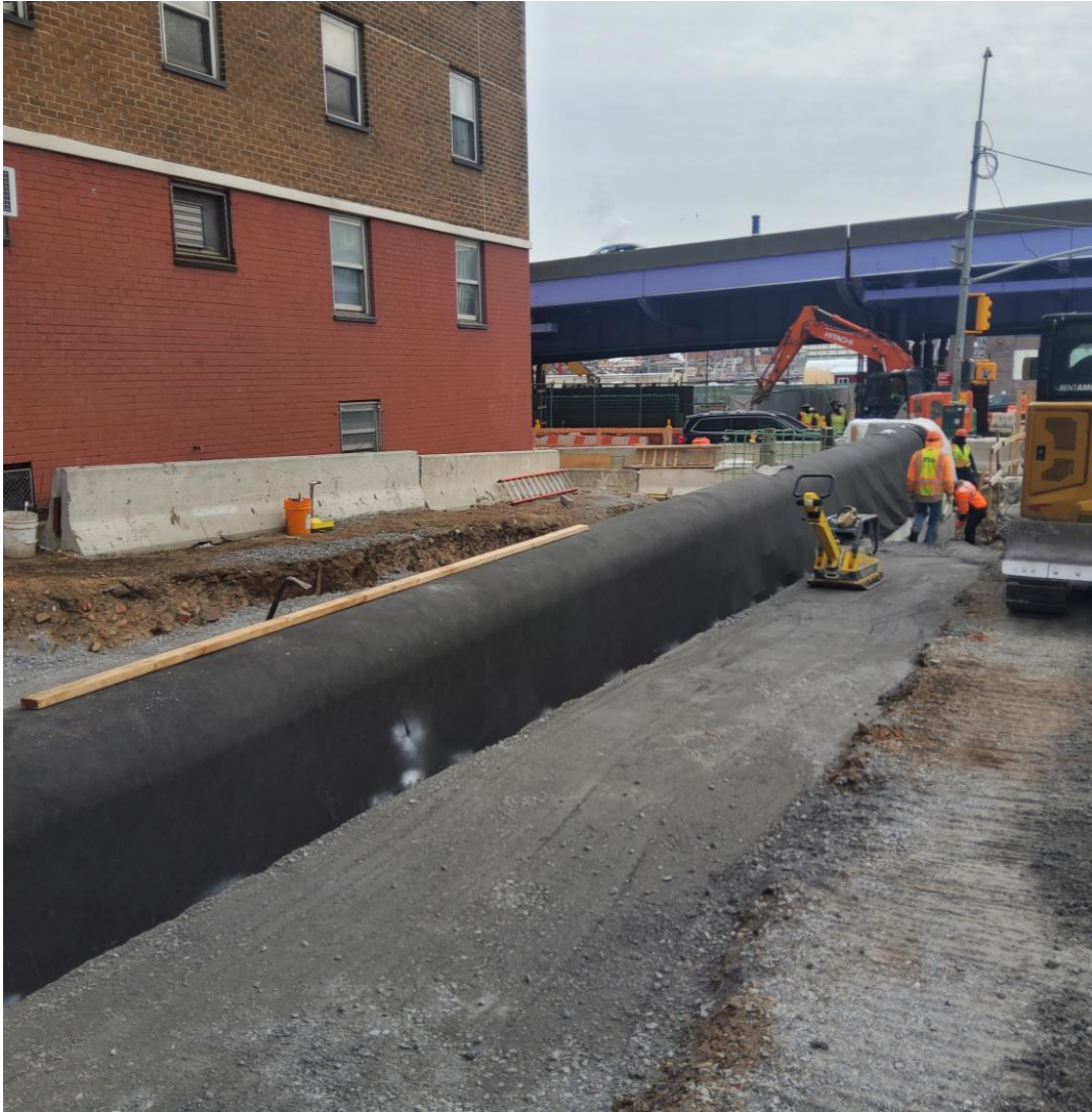
Backfilling floodwall at Montgomery Street and South Street (near Gouverneur Gardens) – January 2025
