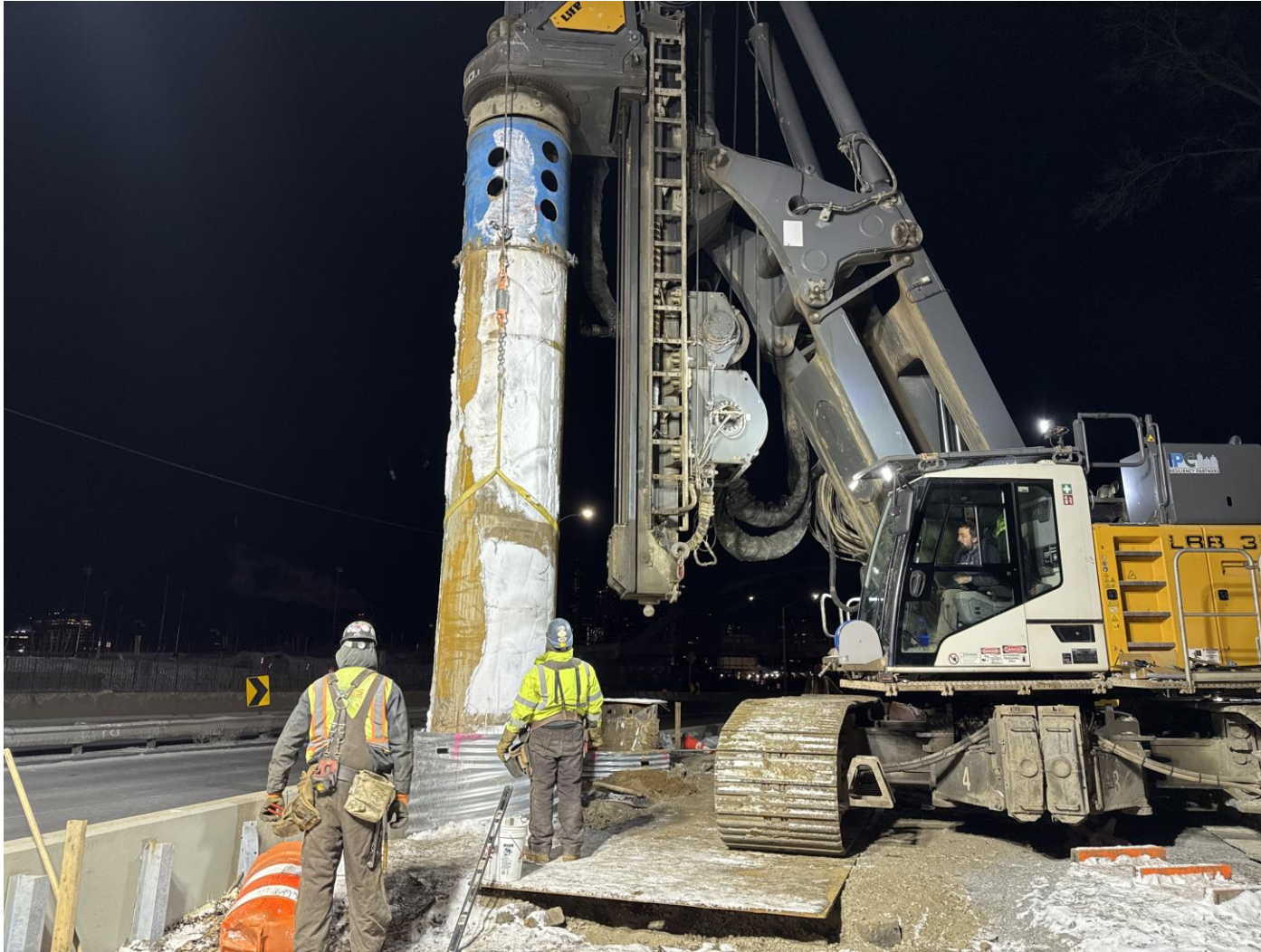
Construction of overhead sign structure shaft near Corlears Hook Park – January 2025
