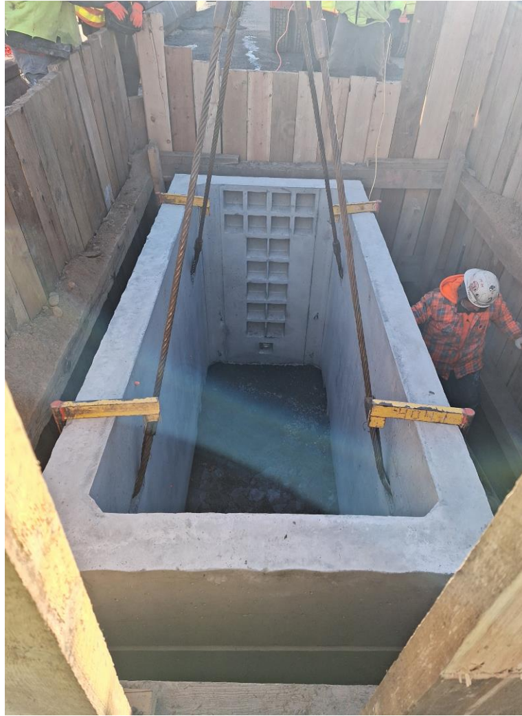
Con Ed manhole installation in E. Houston St. – January 2025
