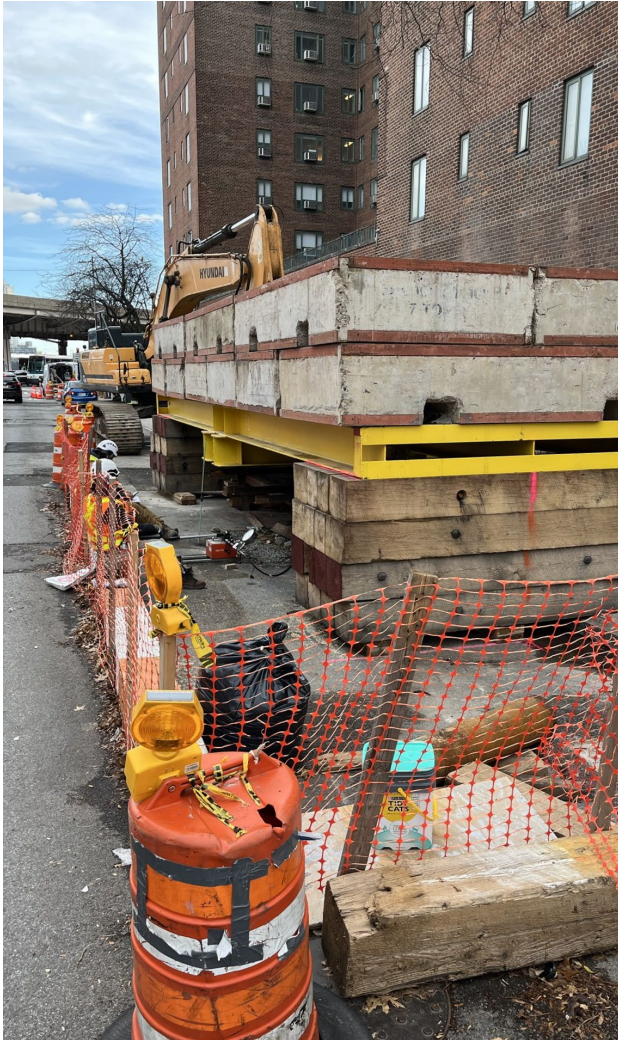
Micropile load test at E. 20 th St. – December 2024
