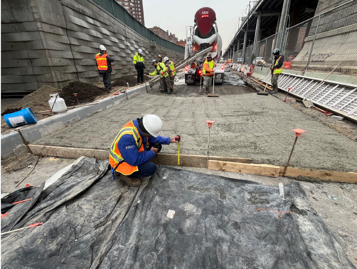
Concrete road base at Delancey Street Pedestrian Bridge – January 2025
