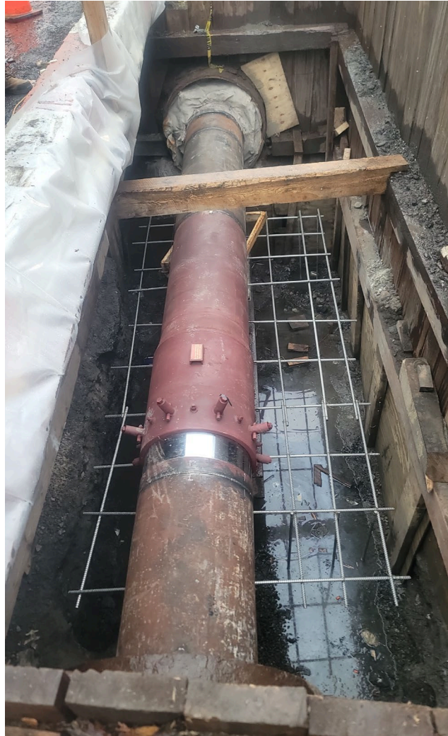
Steam main slip joint at Ave C and E. 18 th Street – December 2024
