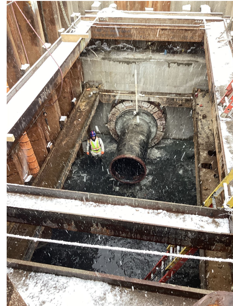
42" sewer pipe installed in launching pit – January 2025
