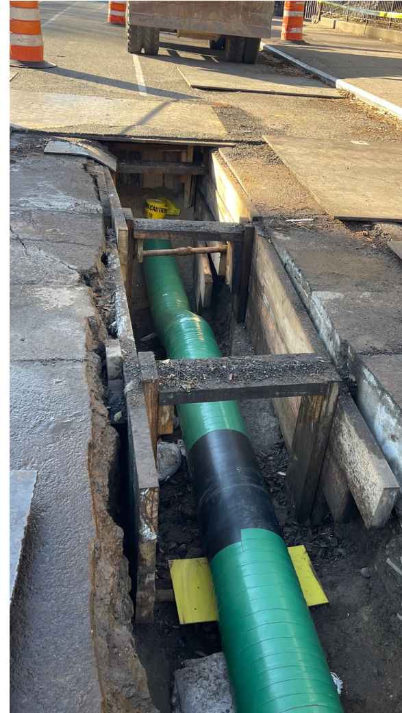
Gas main relocation at E. Houston St. and Columbia St. – December 2024
