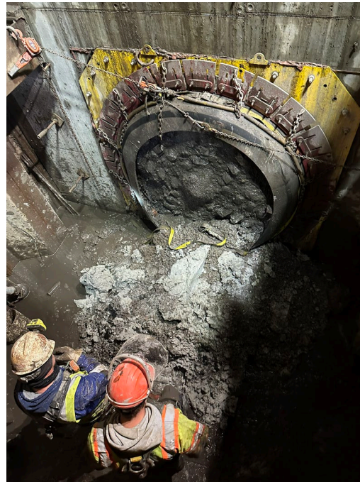
Microtunneling machine breaking through receiving pit – December 2024
