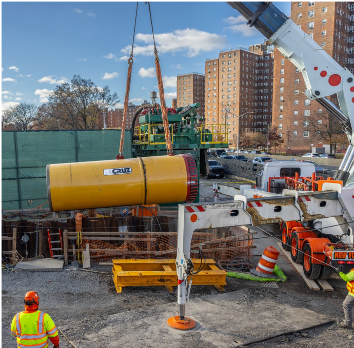
Microtunneling machine lowered into launching pit – December 2024
