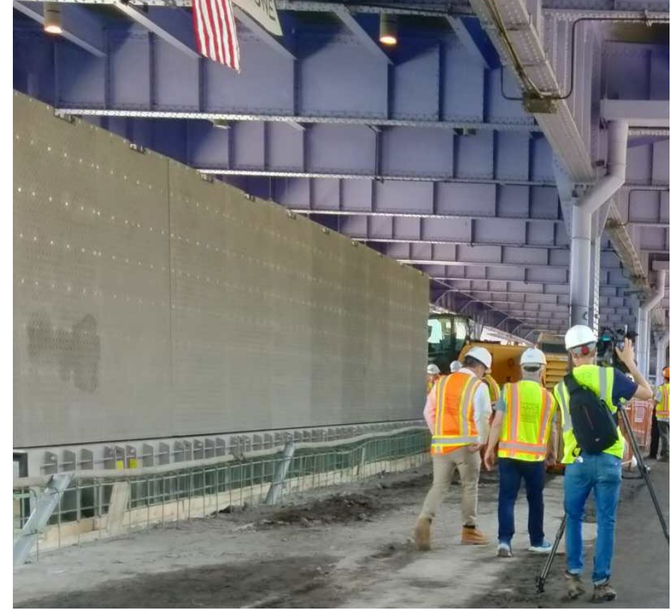
Deployed flip up gate, dry side during installation – June 2024
