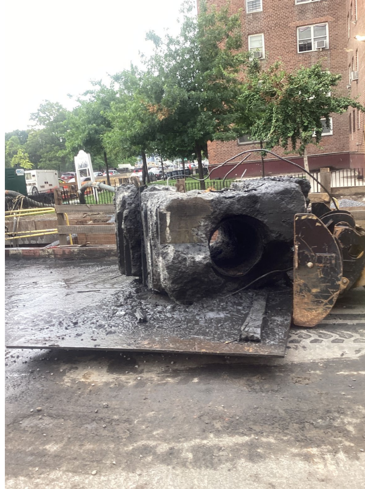
Removal of existing sewer interceptor – July 2024
