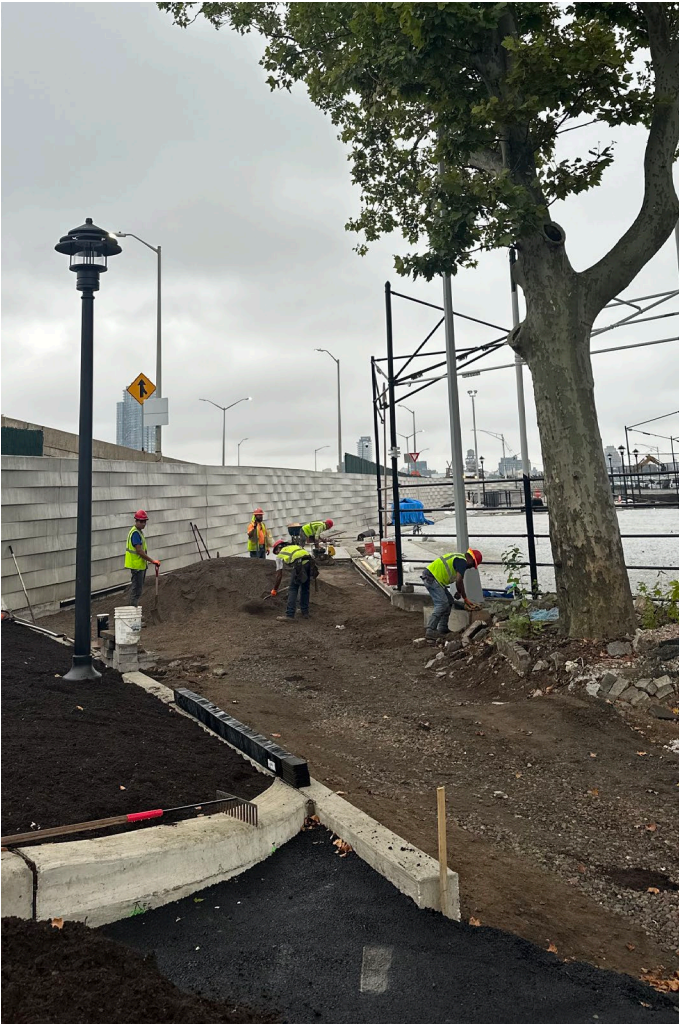
Grading soil for sidewalk – July 2024
