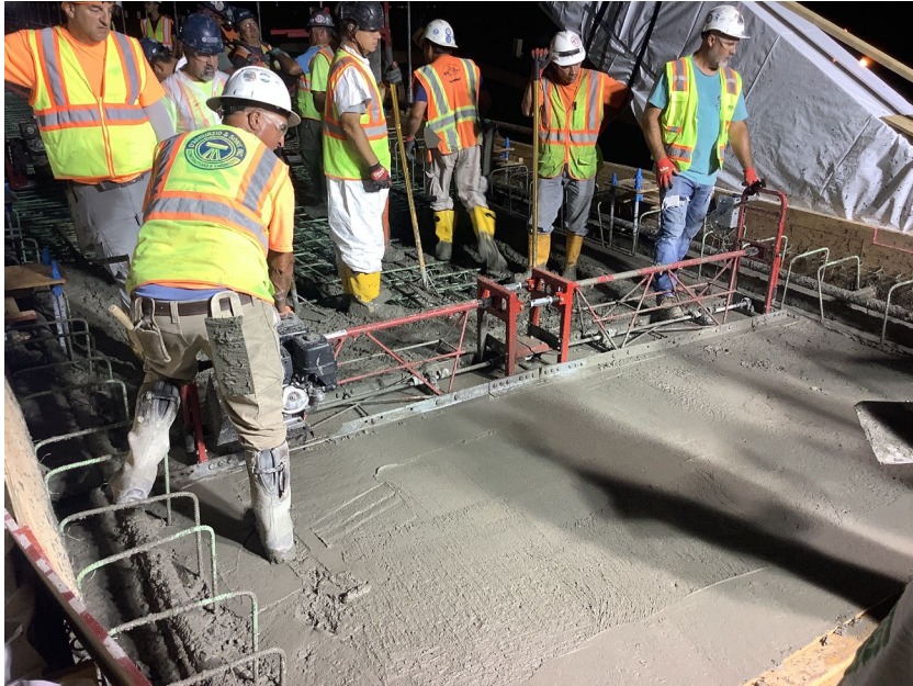
Pouring concrete for Delancey Street Pedestrian Bridge deck – July 2024
