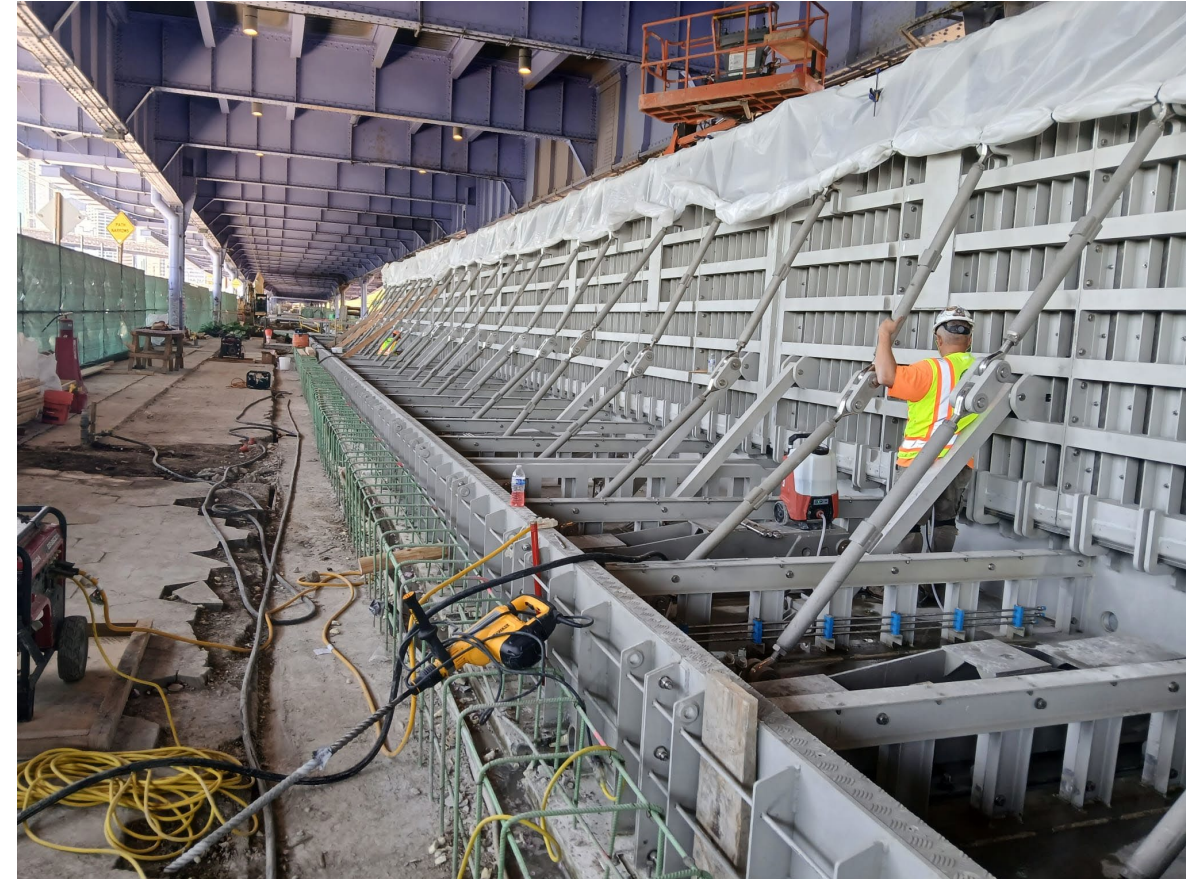
Deployed flip up gate during installation – June 2024
