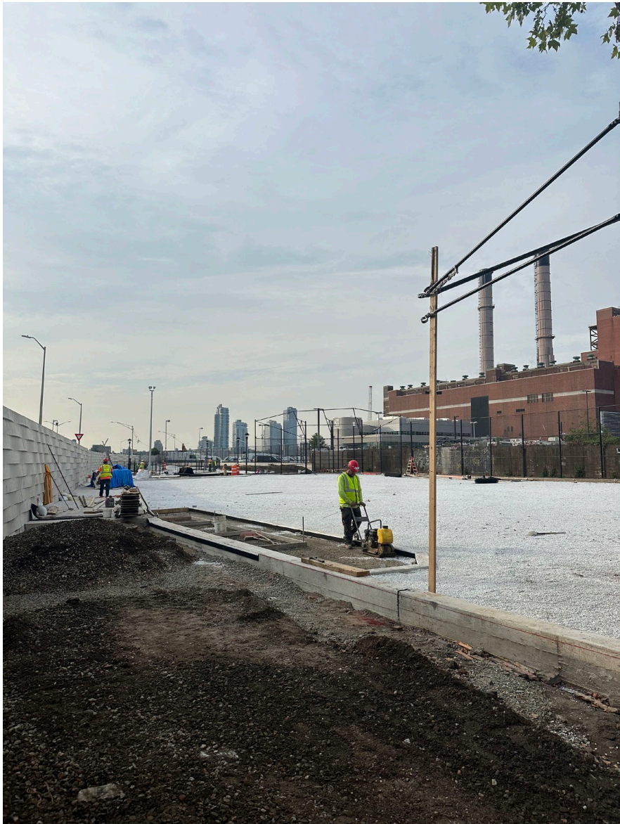
Compacting ground for tee ball dugout – July 2024
