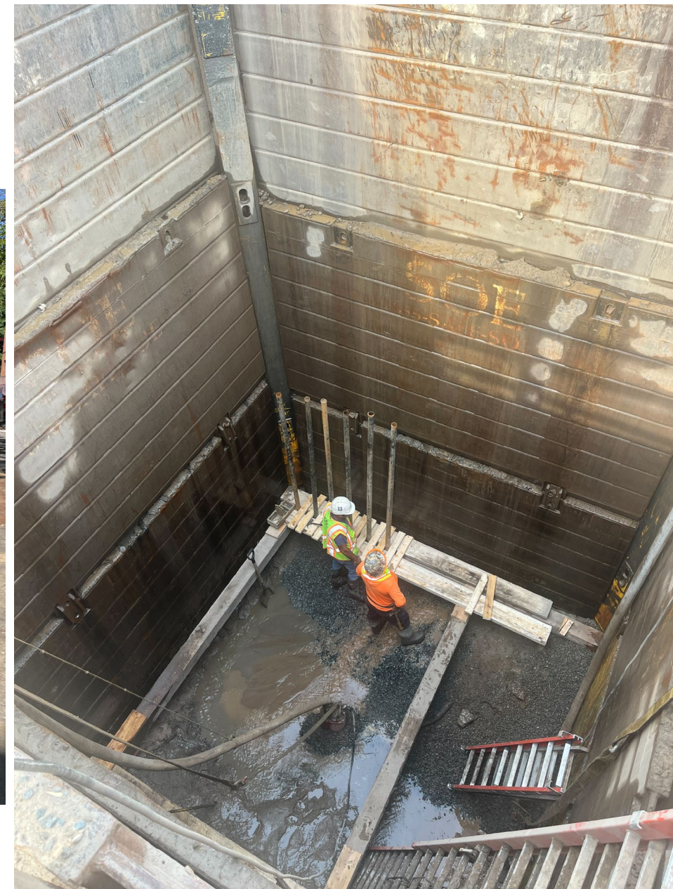
Test pit to locate interceptor sewer – July 2024
