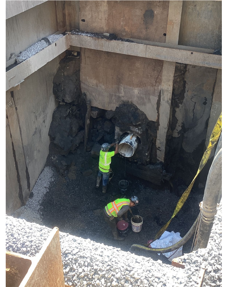
Excavation trench for microtunneling – July 2024
