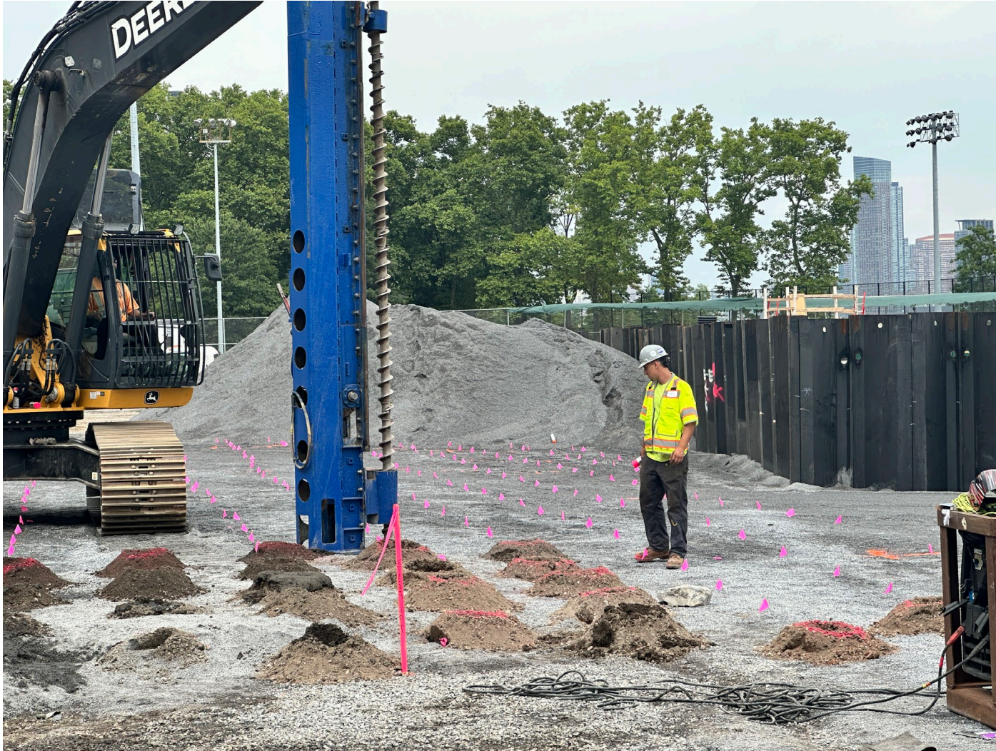
Installation of wick drains near Ballfield 5 – July 2024
