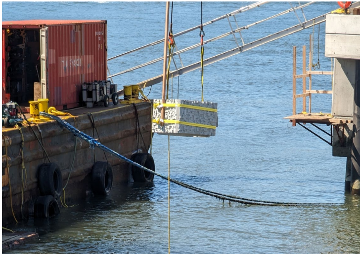
Installation of sea pillars on existing esplanade pipe piles – June 2024
