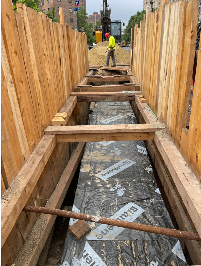
Backfilling ConEd steam main on Columbia St. – June 2024
