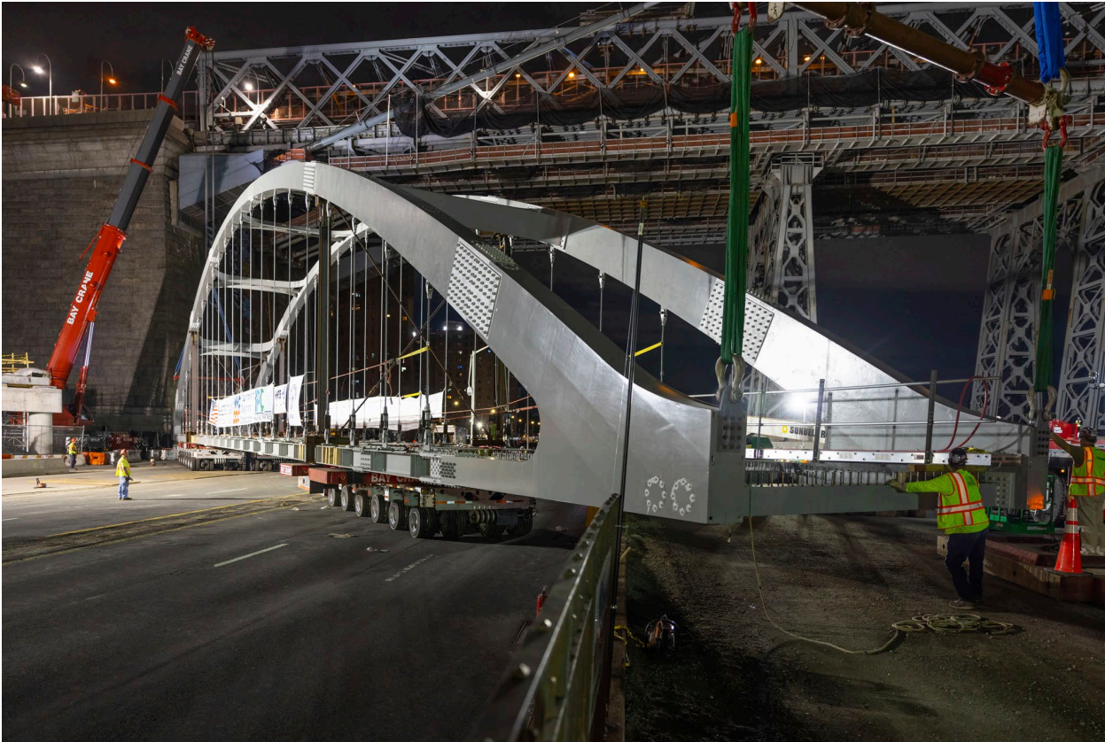
Delancey Pedestrian Bridge on SPMT transporters at installation location just south of the Williamsburg Bridge – June 2024
