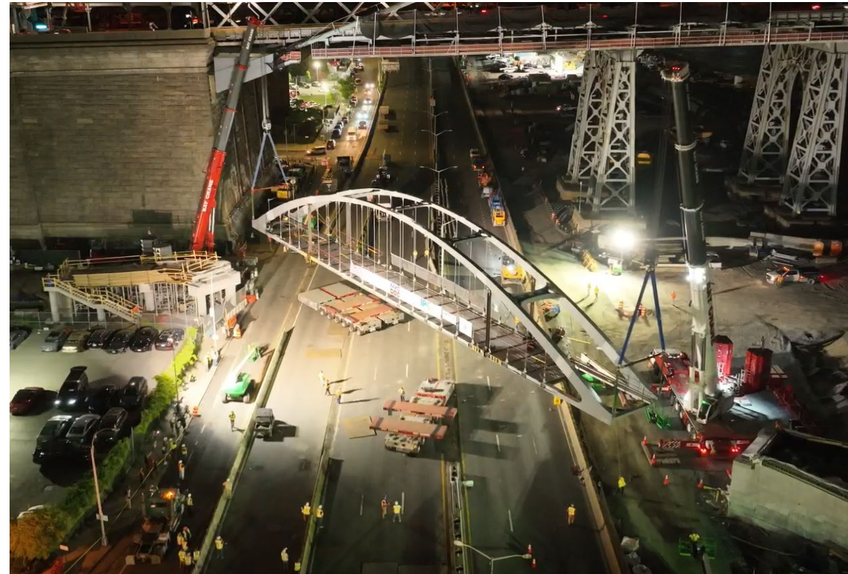
Delancey Pedestrian Bridge lifted by two cranes into place – June 2024
