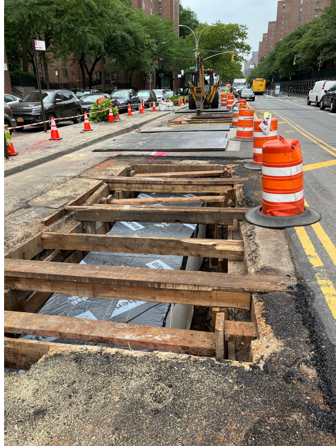
ConEd steam main encasement on E 20 th St. between Ave C and E. 20 th St. loop – June 2024
