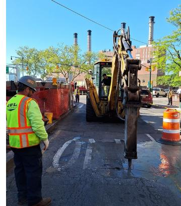
Test Pit to locate Steam main bend at E 18th St and Ave C intersection – May 2024
