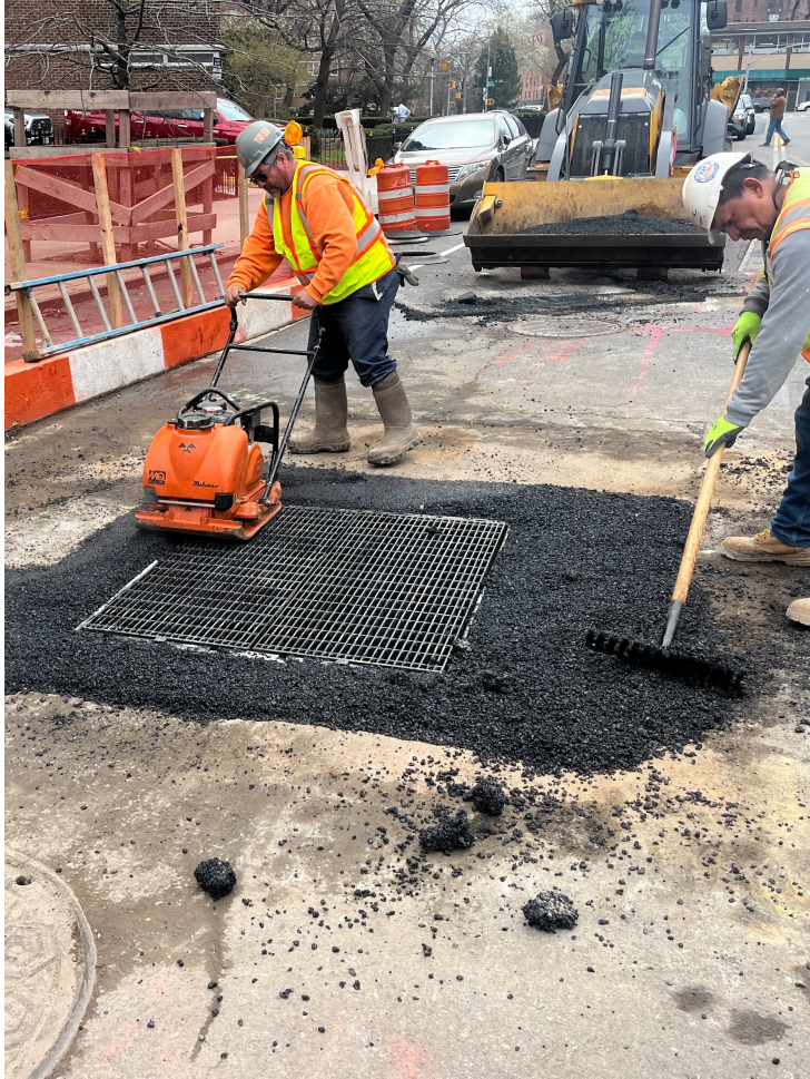
Installation of Con Ed manhole casting Lewis - April 2024
