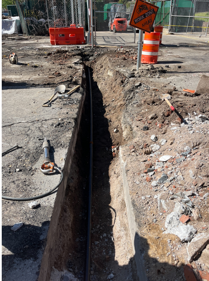
Streetlight conduit installation Delancey and Baruch Dr - April 2024
