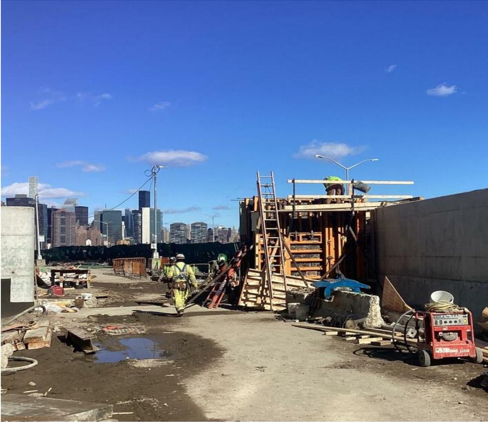
*Flood Gate 8 east column formwork – February 2024*
