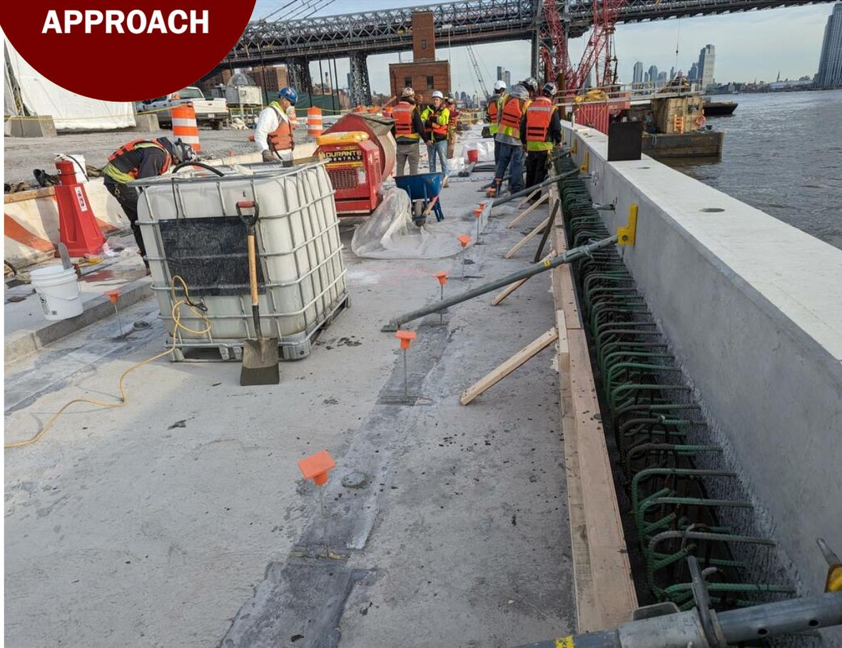
*Esplanade Construction: sloped parapet installation – February 2024*
