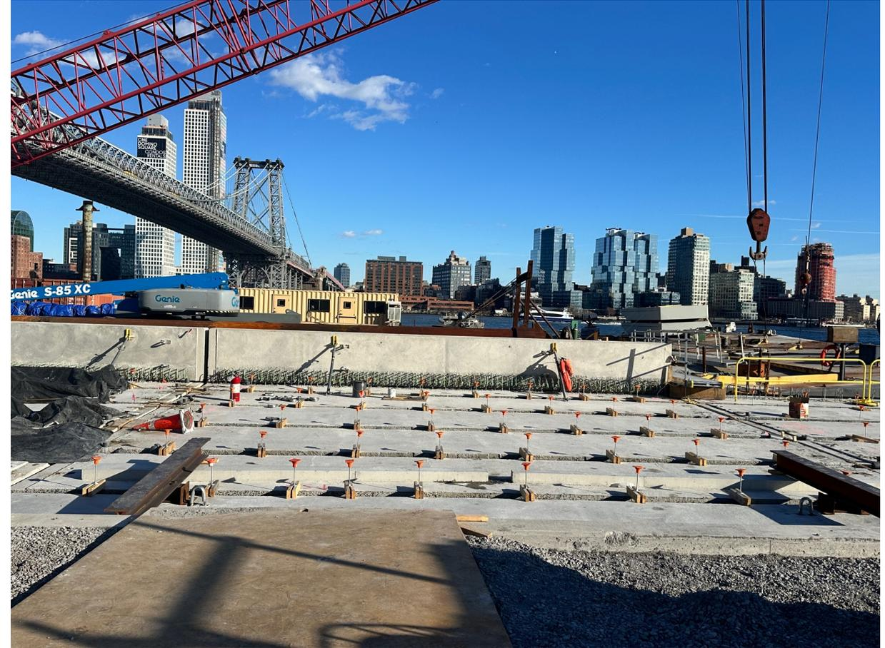
*Esplanade Construction: sloped parapet installation – February 2024*
