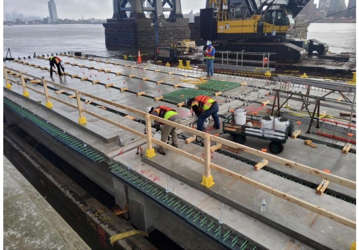
*Prefabricated esplanade support beams in place - January 2024*
