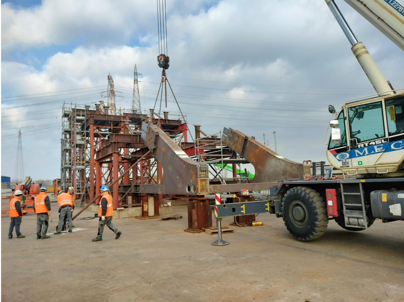
*Test fit of Delancey Street Bridge superstructure at fabrication facility - November 2023*
