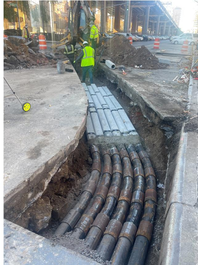
ConEd ducts installation in Delancey St. North by
