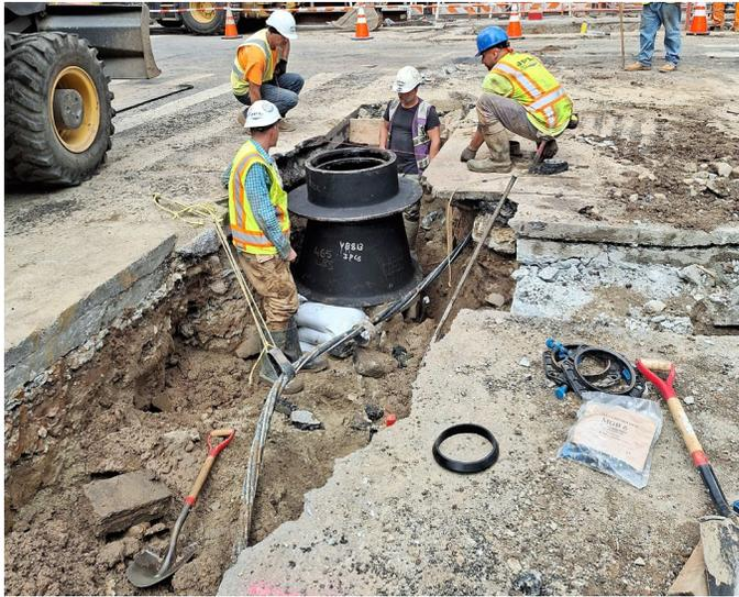
*Casting water main valve on Gouverneur Slip E.
