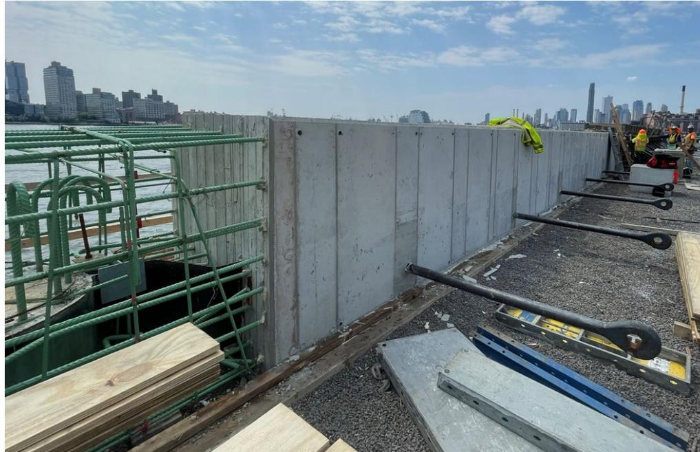
3. Rebar box cage is constructed on-site and installed over piles.
