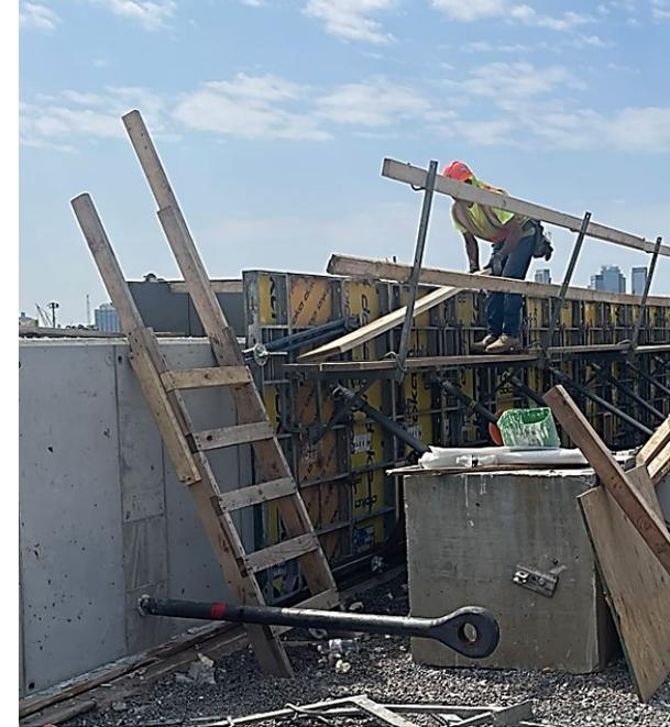
4. Wood forms are placed, and concrete is poured to create Cap Wall.
