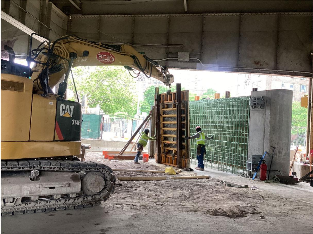
Installing formwork E 18<sup>th</sup> Street (Gate 10 & 11) - May 2023
