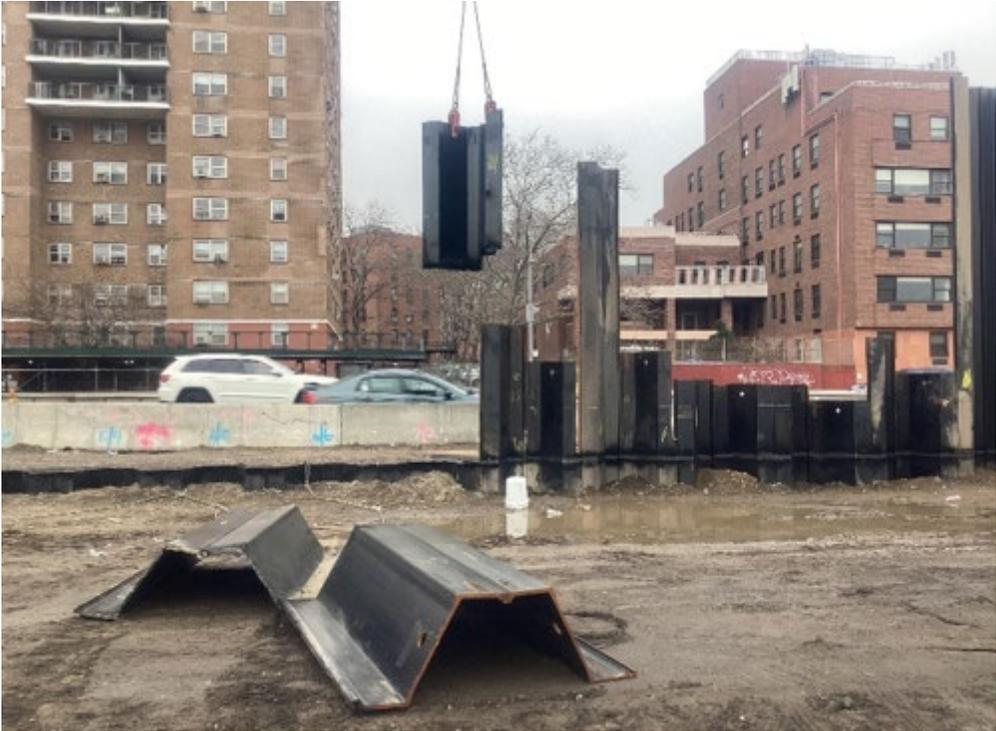
Montgomery Greenway Floodwall Sheet Pile installation complete as of January 2023
