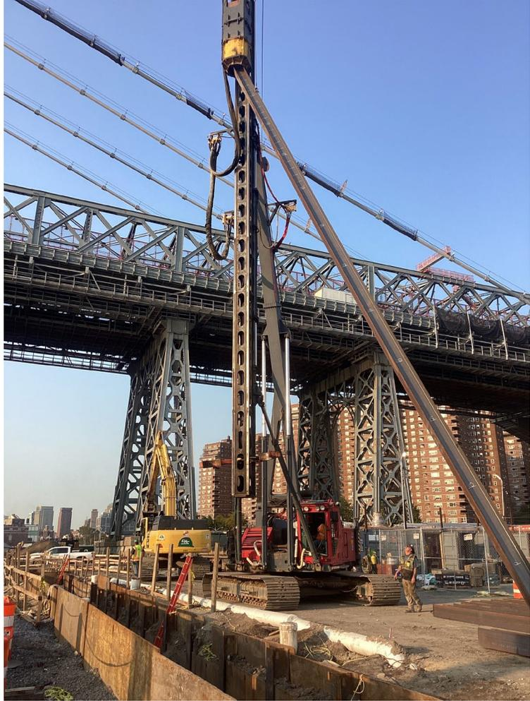
*H-pile installation for deep sewer work – September 2022*
