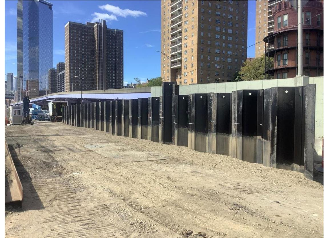
*Sheet Pile installation for floodwall along the Greenway with vibrating pile rig – September 2022*
