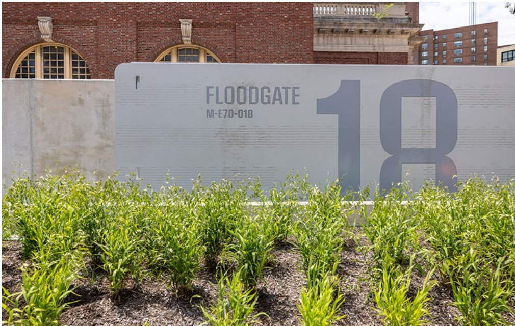
Asser Levy Playground Floodgate #18 – July 2022
