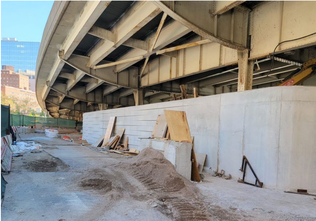
Floodwall under FDR Dr. at E 23 rd Street – July 2022
