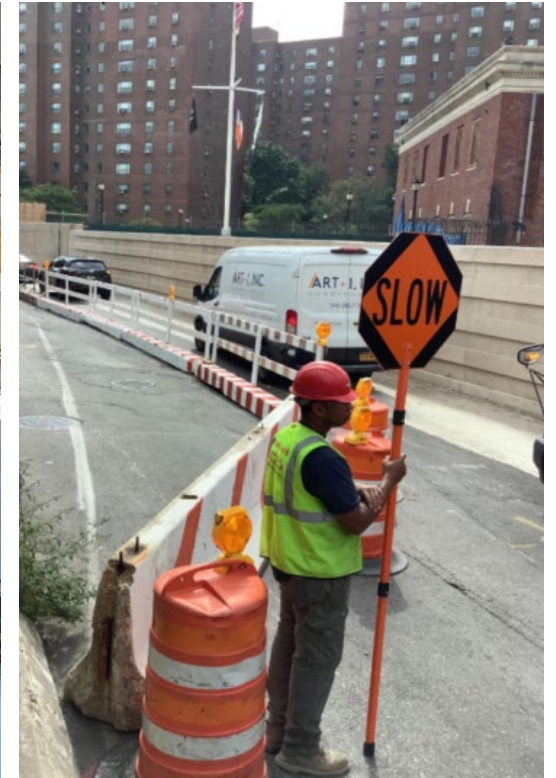
Floodwall along West Service Road – Sept '22
