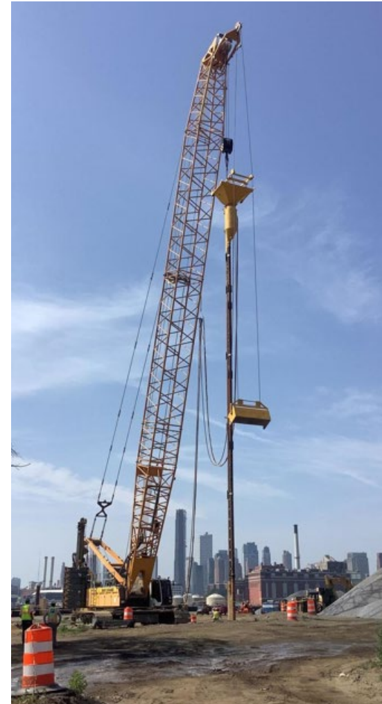
Prepping for stone load – July 2022
