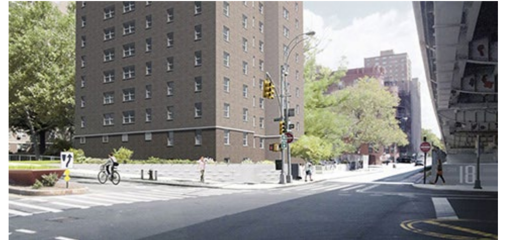
Montgomery St. / South St. floodwall and flood gate
