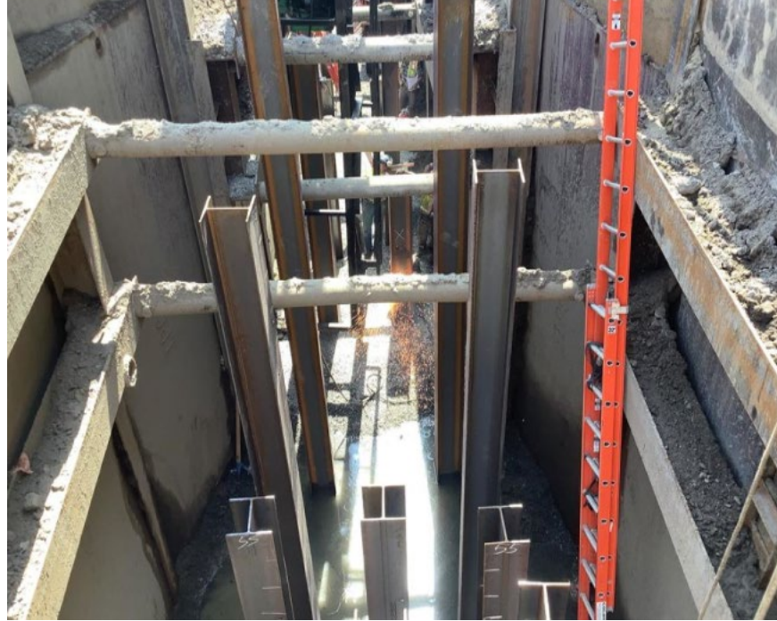
H-Pile install - July
