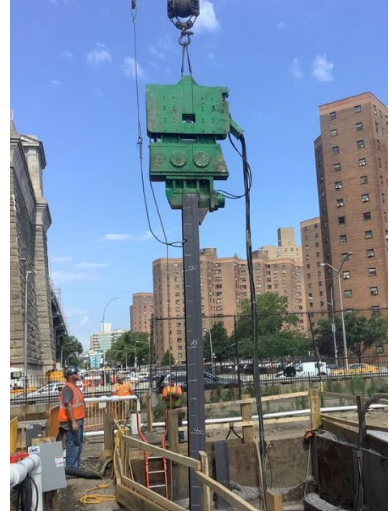
H-Pile install with vibratory hammer - July
