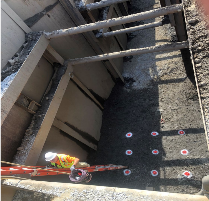
Shoring and markers for H-Pile install – red dots indicate locations of H-Piles - June
