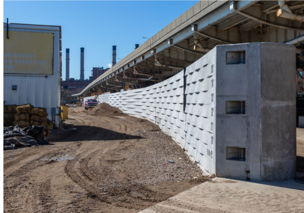
Stuyvesant Cove Park floodwall with elevation markings May 2022
