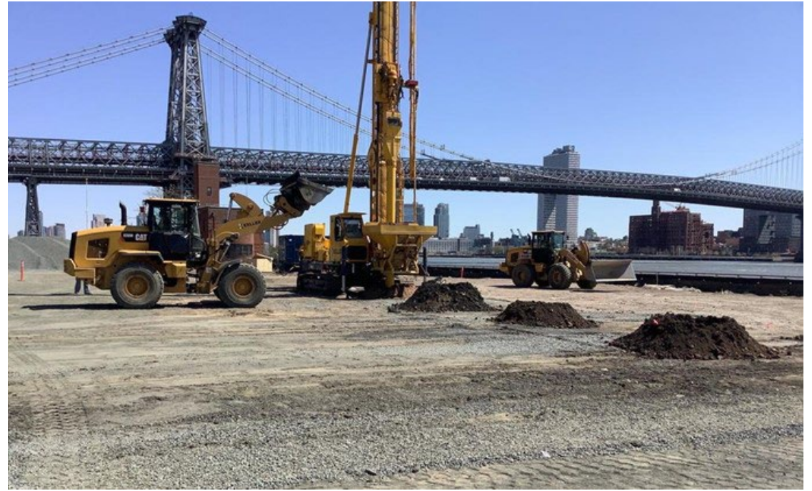
#1 Esplanade Soil Stabilization in progress May 2022
