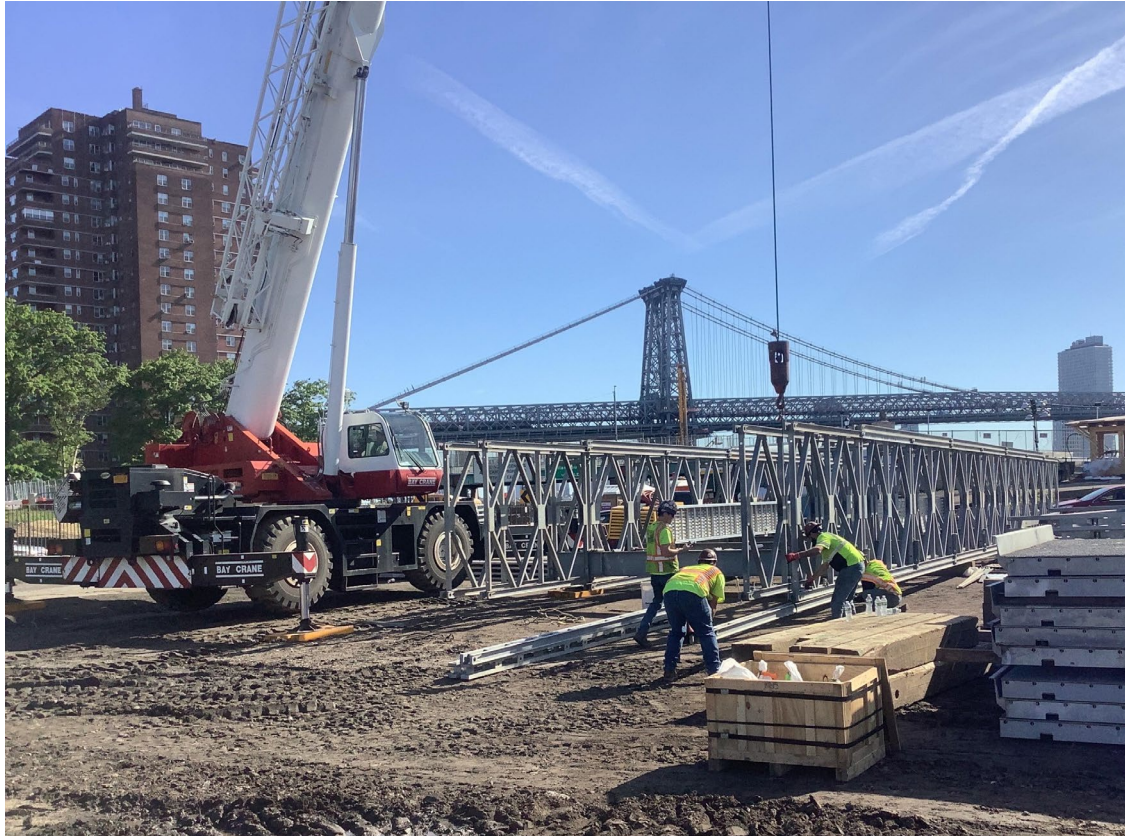
#3 Corlears Hook Temporary Pedestrian Bridge assembly in progress May 2022
