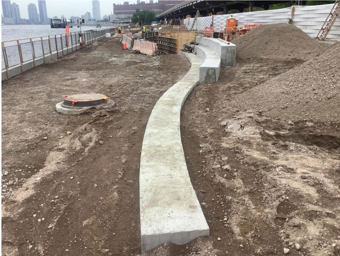
Stuyvesant Cove Park seat wall in progress May 2022
