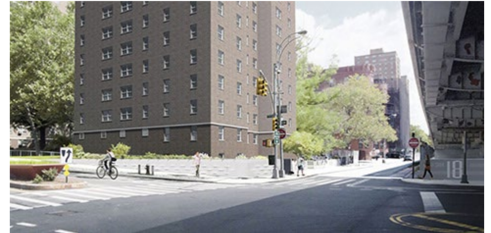
#6 Montgomery St. / South St. floodwall and flood gate
