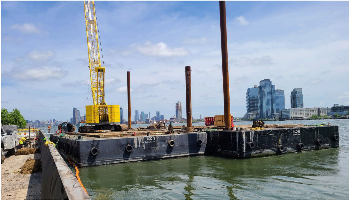
#1 Barges and Crane arrives
