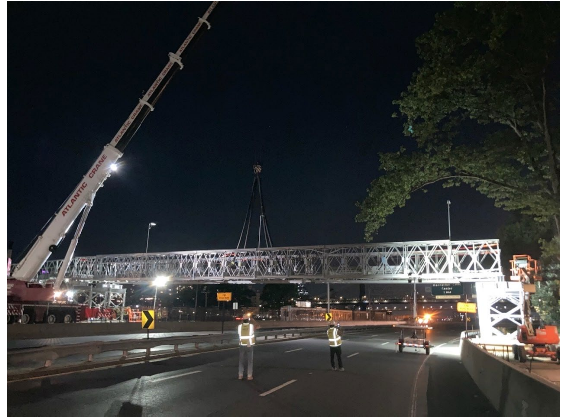
#3 Corlears Hook Temporary Pedestrian Bridge install June 5, 2022
