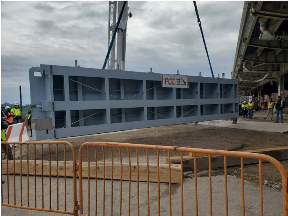
Stuyvesant Cove Park Vehicular Swing Gate install 2/24/2022
