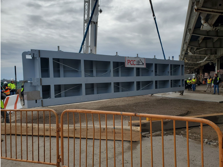
Stuyvesant Cove Park Vehicular Swing Gate install 2/24/2022
