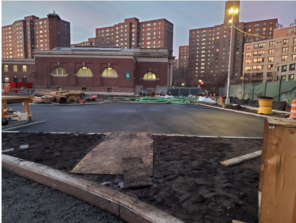
Asser Levy Playground reconstruction (looking south)
