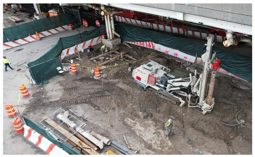
Micro pile installation: intersection of E 23<sup>rd</sup> Street and Avenue C adjacent to BP Gas Station (July 2021)
