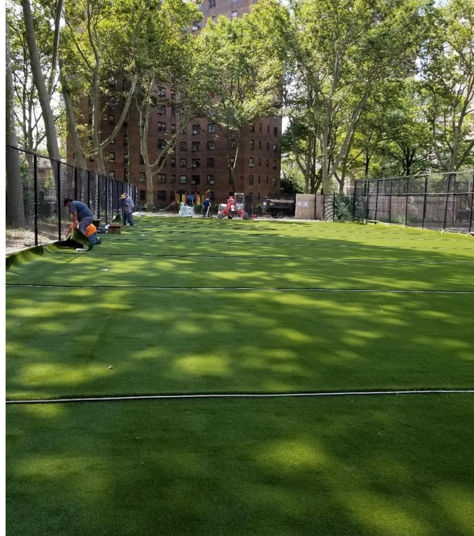
LaGuardia Bath House Demolition/Turf Installation
