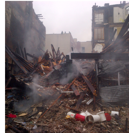
GAS EXPLOSION IN EAST HARLEM 2014
