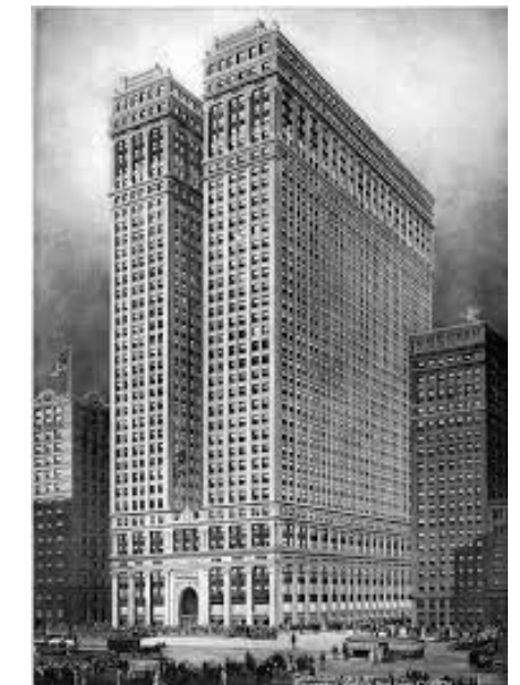
42-STORY EQUITABLE BUILDING 1915
