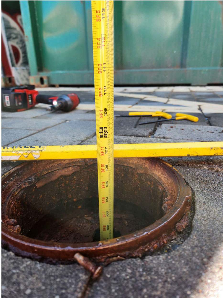
Photo 4 – Inspection Port on Pier Deck
