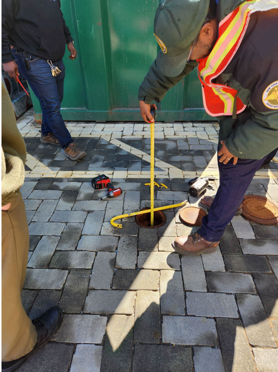
Photo 5 – Inspection Port on Pier Deck
