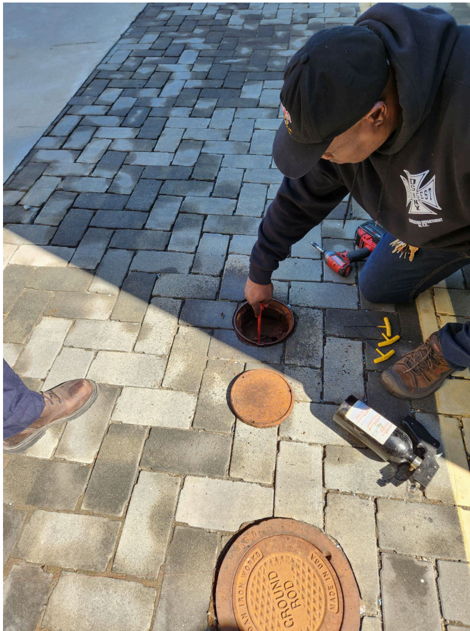
Photo 2 – Measurement Tape Lowered into Inspection Port
