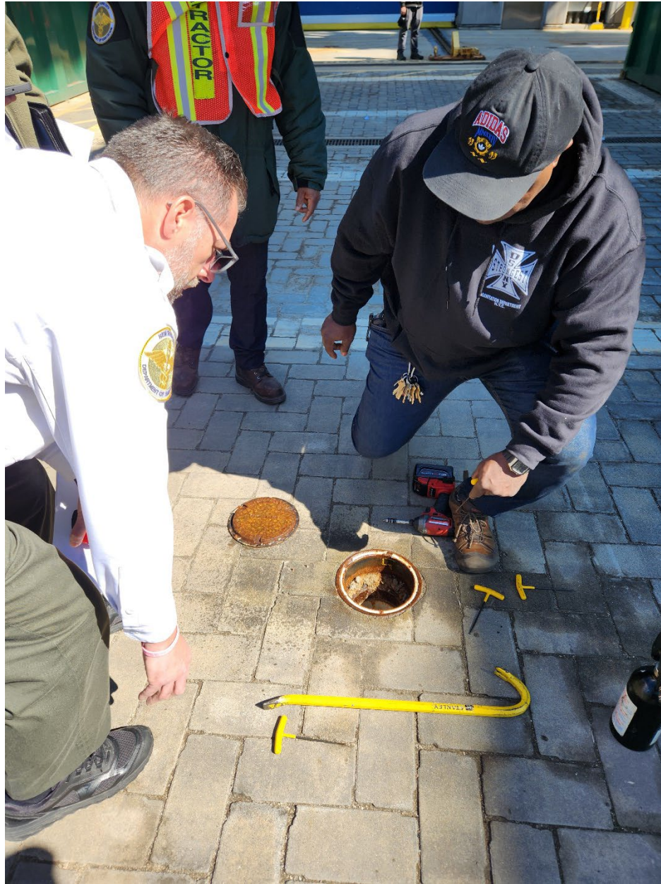
Photo 1 – Inspection Port on the Pier Deck
