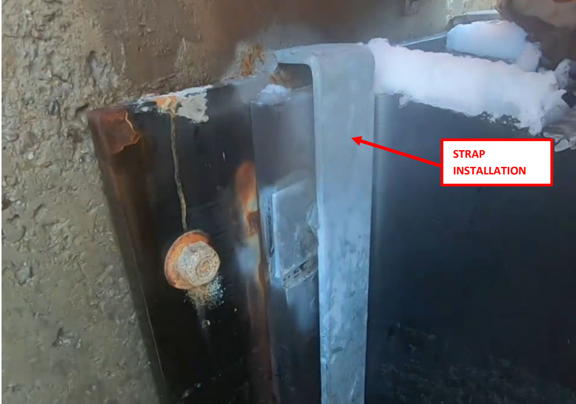
Photo 3: Typical strap repair.
