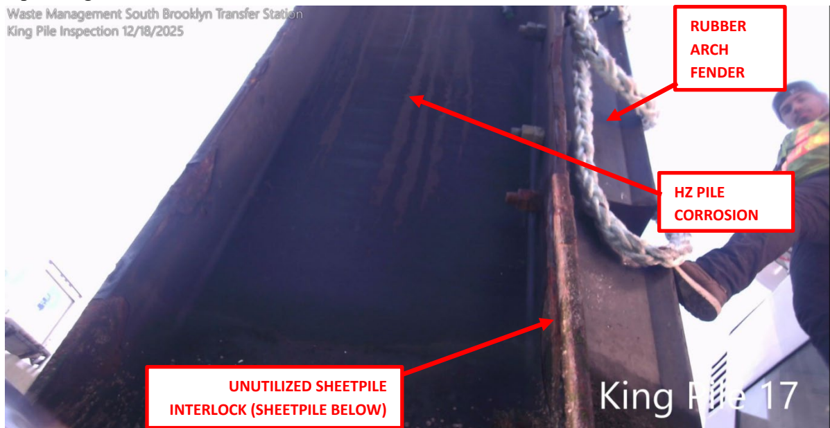
Photo 18: Typical condition of King Pile.
