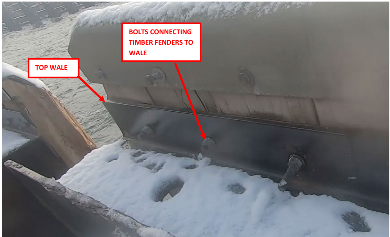
Photo 9: Typical Condition of top Wale.
