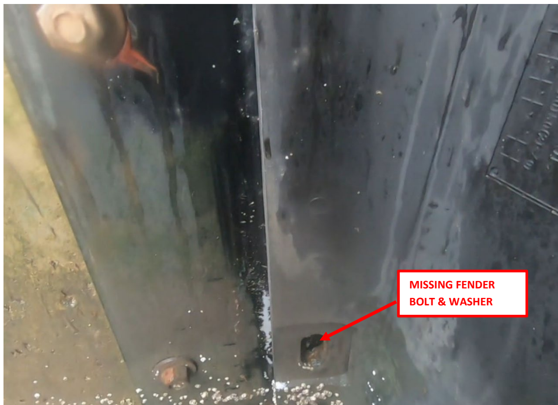
Photo 2: Rubber fender bolt connecting fender to mounting plate.
