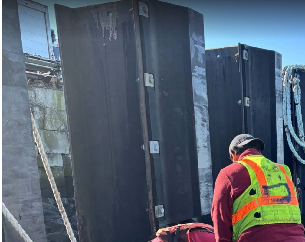
Photo 20: Typical condition of Upper Rubber Arch Fender.
