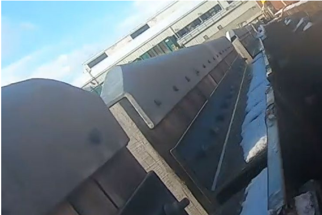
Photo 12: Typical Condition of fender timbers from interior side.
