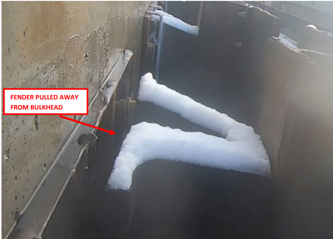
Photo 1: Rubber fender separated from mounting plate w/ top 2 bolts pulling out of fender.
