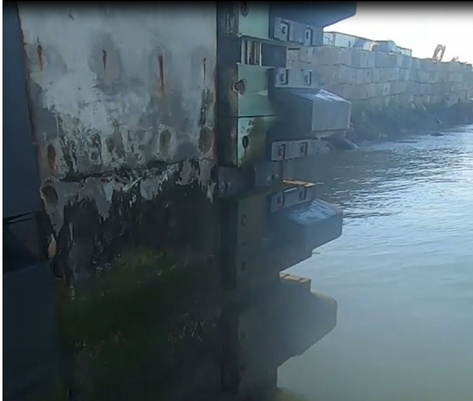
Photo 24: Above-water condition of End Fender.
