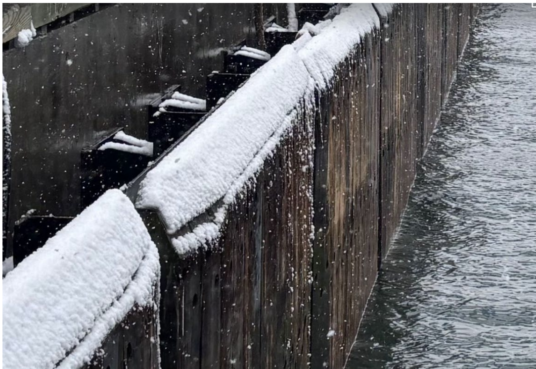
Photo 13: Typical Condition of fender timbers from exterior side
