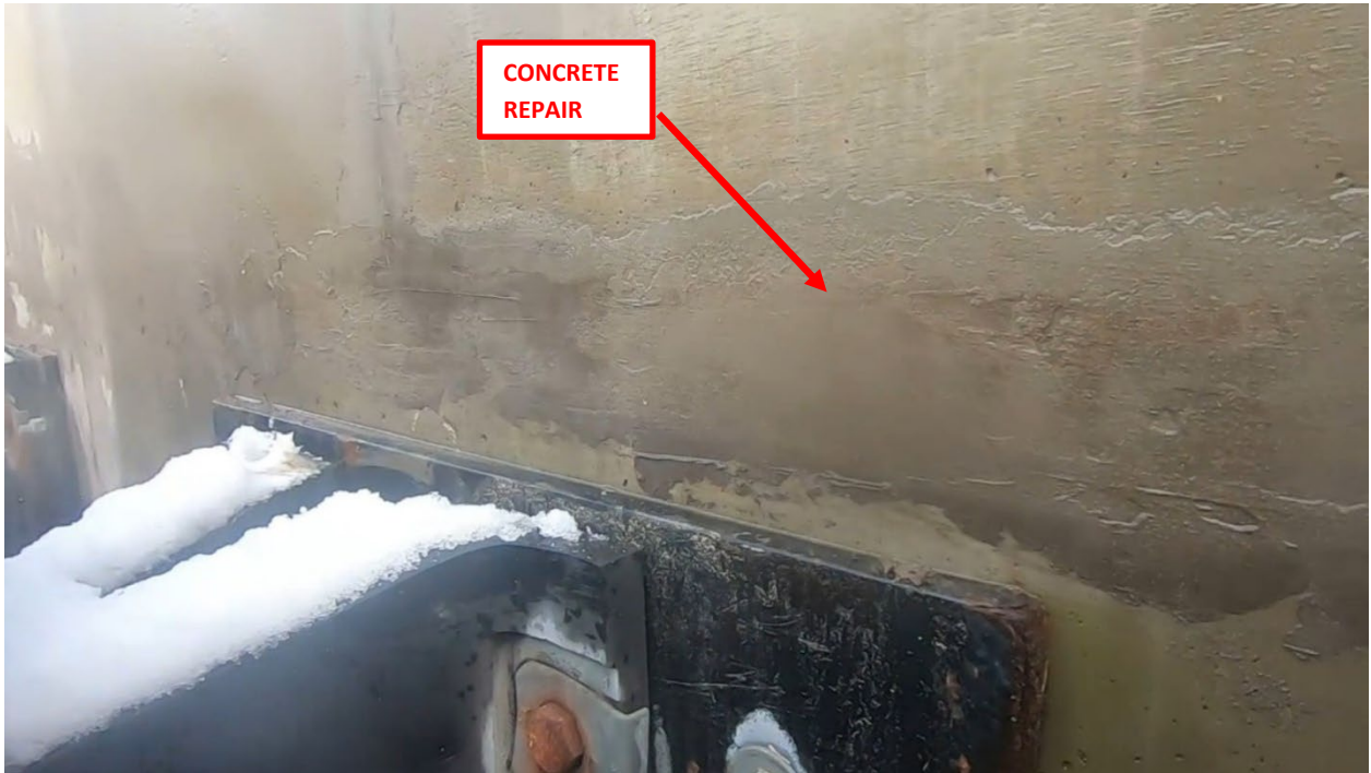
Photo 14: Typical concrete seawall repairs.
