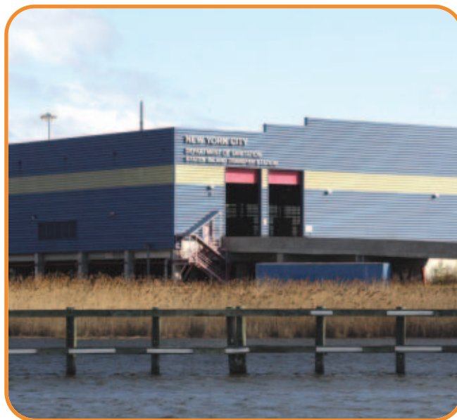
STATEN ISLAND TRANSFER STATION
