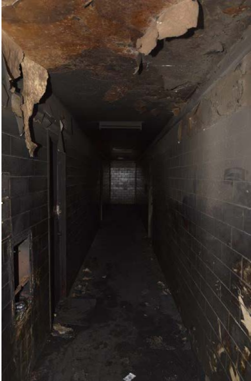
Charred hallway with missing hopper door, and compactor chute with fire damage to hopper door; building B1, Mitchell Houses. Photos courtesy of FDNY BFI.
