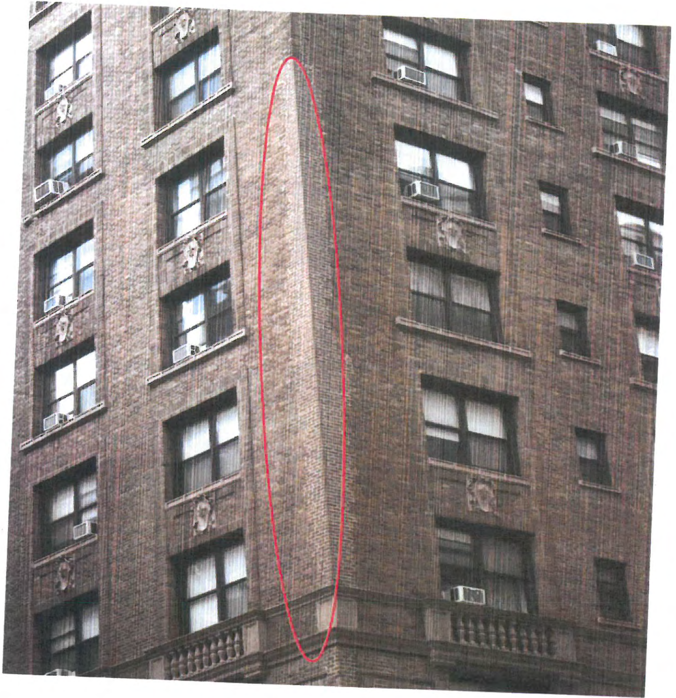
New Repointing of Mortar Joints
