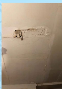
Pictured: Roof Repairs
