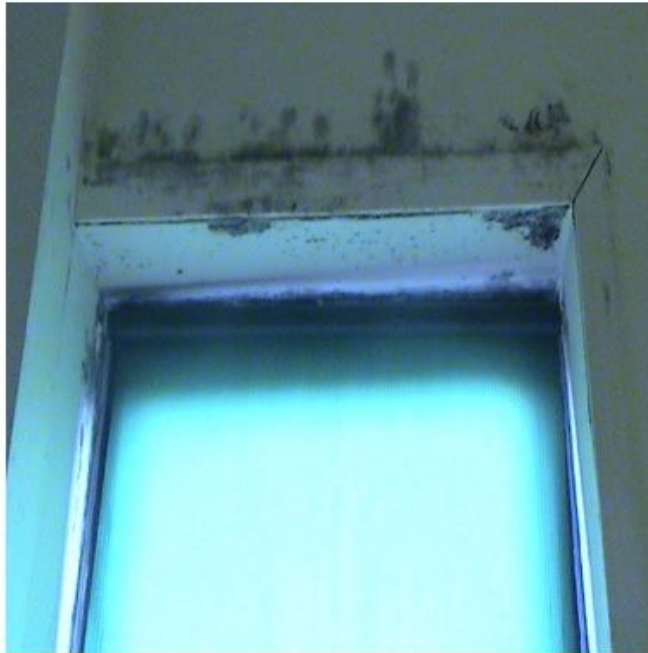
Figure 7: Mike's House (hotel): A 5th floor apartment. Evidence of mold in the bathroom (left): exposed heating pipe in the resident's children's room (right). The exposed portion would be reachable by the children (ages 3, 5, and 7).
