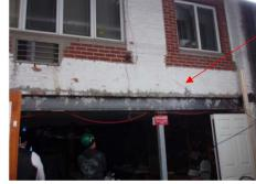
CRACK IN EXTERIOR FAÇADE COMPROMISING STRUCTURAL INTEGRITY AND IN DANGER OF A COLLAPSE
