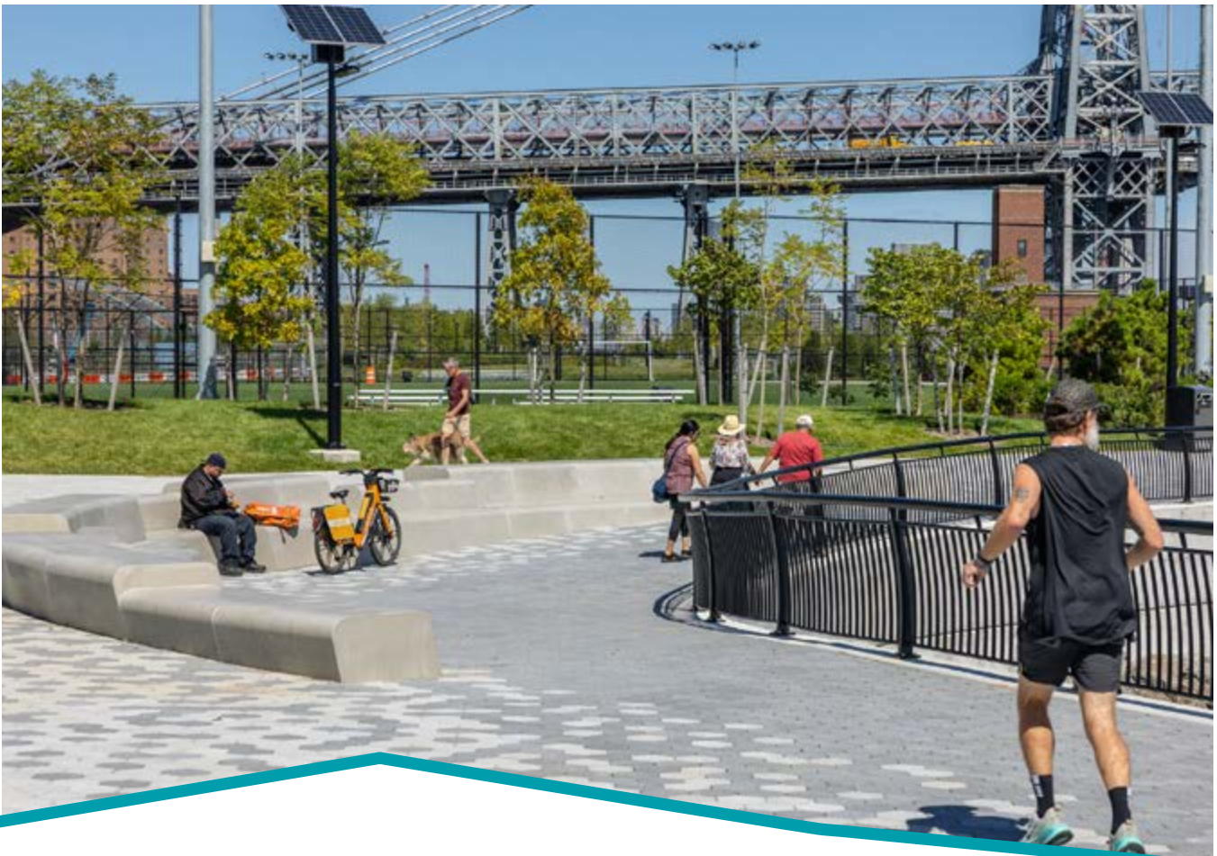
Above: East River Park, Manhattan. To protect New Yorkers from coastal flooding, the East Side Coastal Resiliency Project raises the park by eight feet. (NYC: DDC, Parks, DEP, DOT; Project Team: AKRF-KSE, MNLA, BIG, ONE Architecture and Urbanism)
