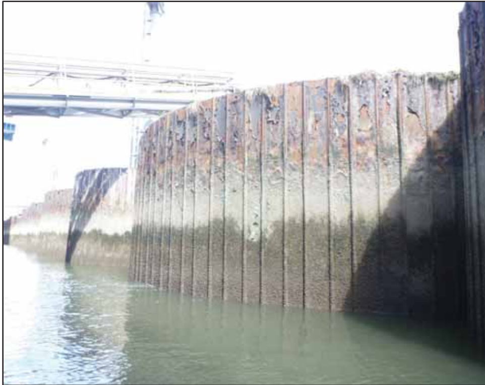
Photo 37-Bulkhead on south side looking west
