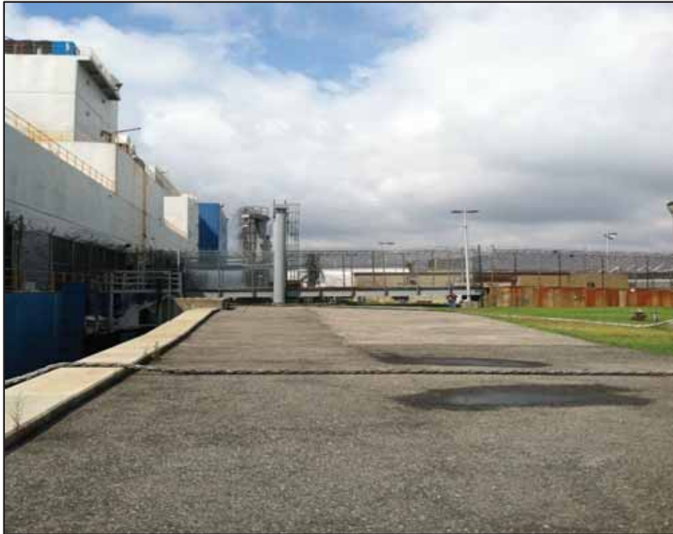
Photo 29-Typical platform area at east end looking west
