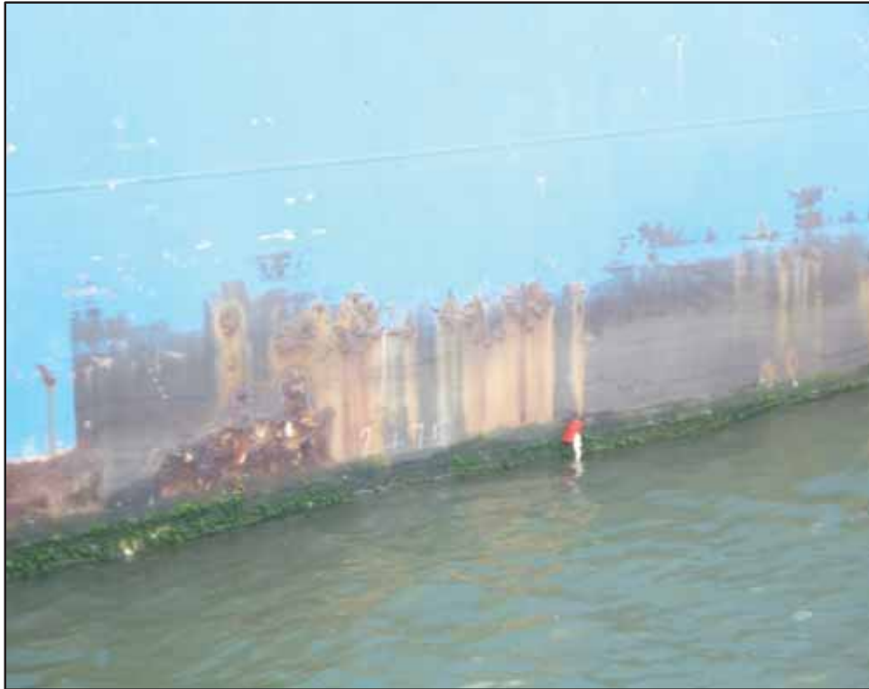
Photo 45-Coating loss in splash zone at Station 2 + 75 on south side
