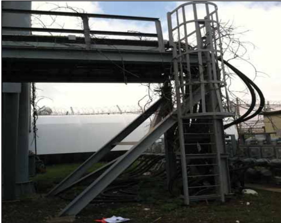
Photo 17-Landside connection of utility gangway at Station 7 + 53
