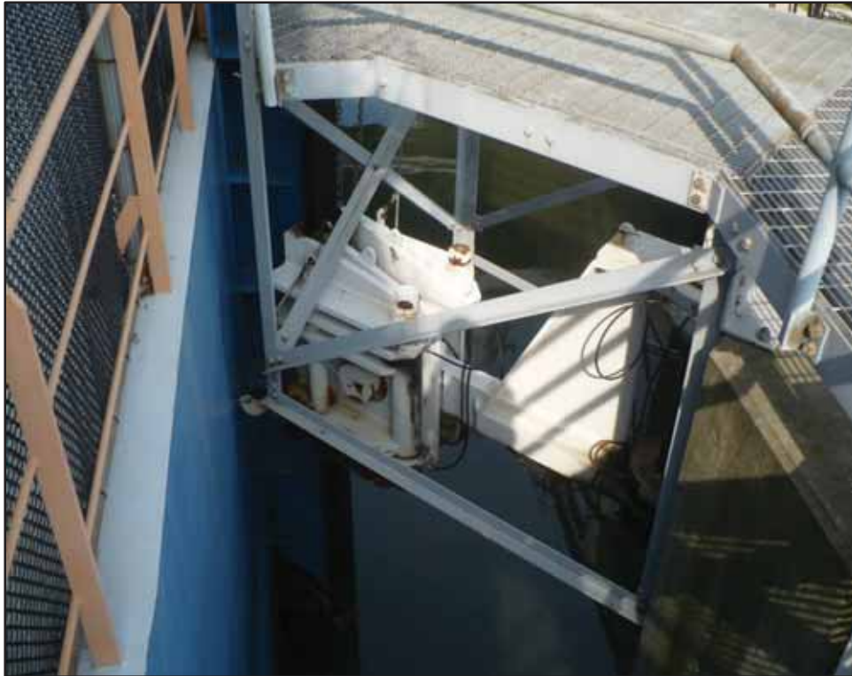
Photo 23-Double mooring barge side connection at Station 8 + 32
