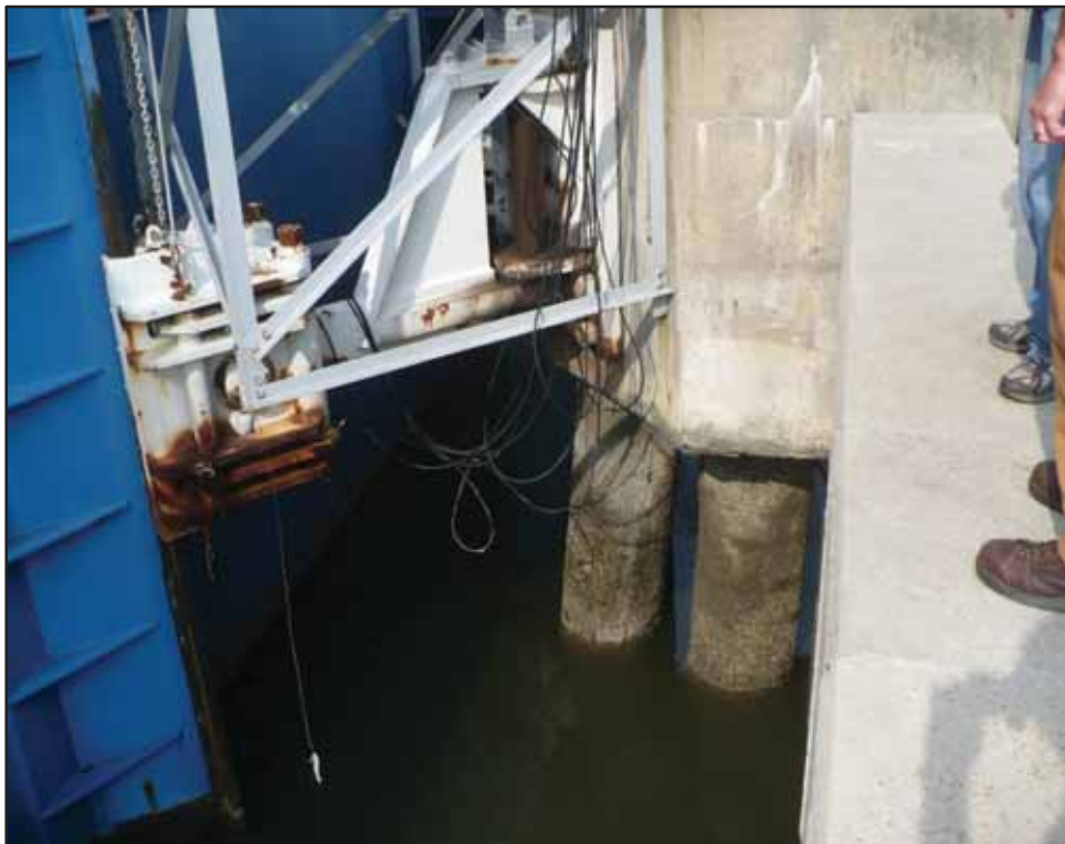
Photo 22-Double mooring landside connection at Station 8 + 32
