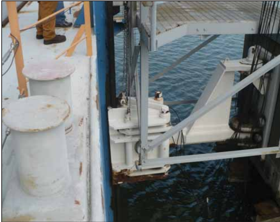
Photo 7-Single mooring connection at Station 3 + 22 looking west
