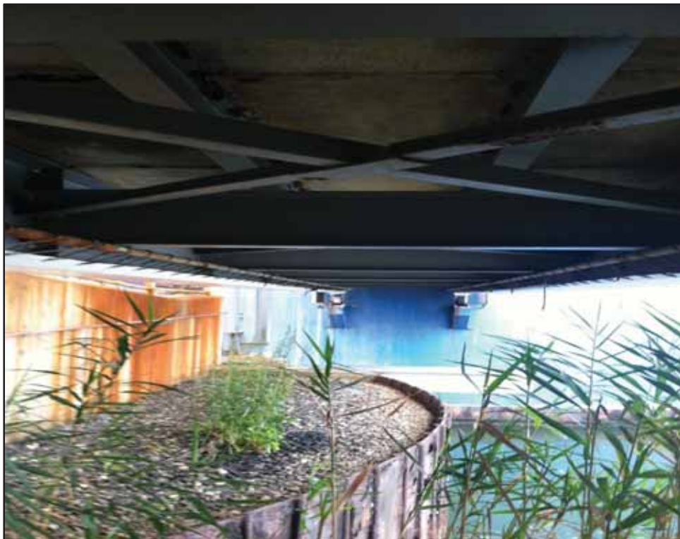
Photo 4-Underdeck of gangway at Station 3 + 10
