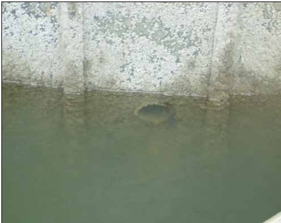
Photo 40-Submerged pipe on west side of bulkhead through Sheet 11 of Cell 14
