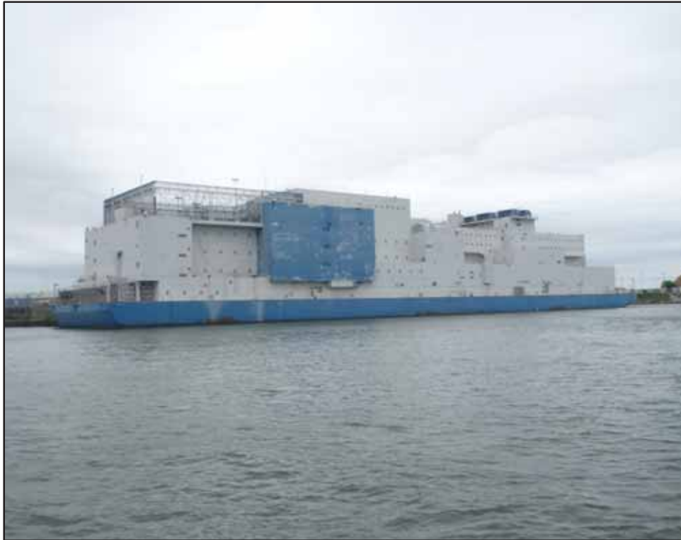
Photo 1-Overall photo of VCBC looking north
