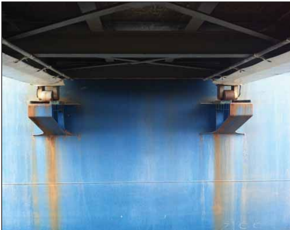
Photo 10-Underdeck and rollers of gangway at Station 4 + 90
