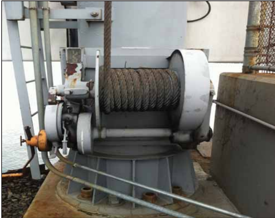
Photo 5-Winch of gangway at Station 3 + 15
