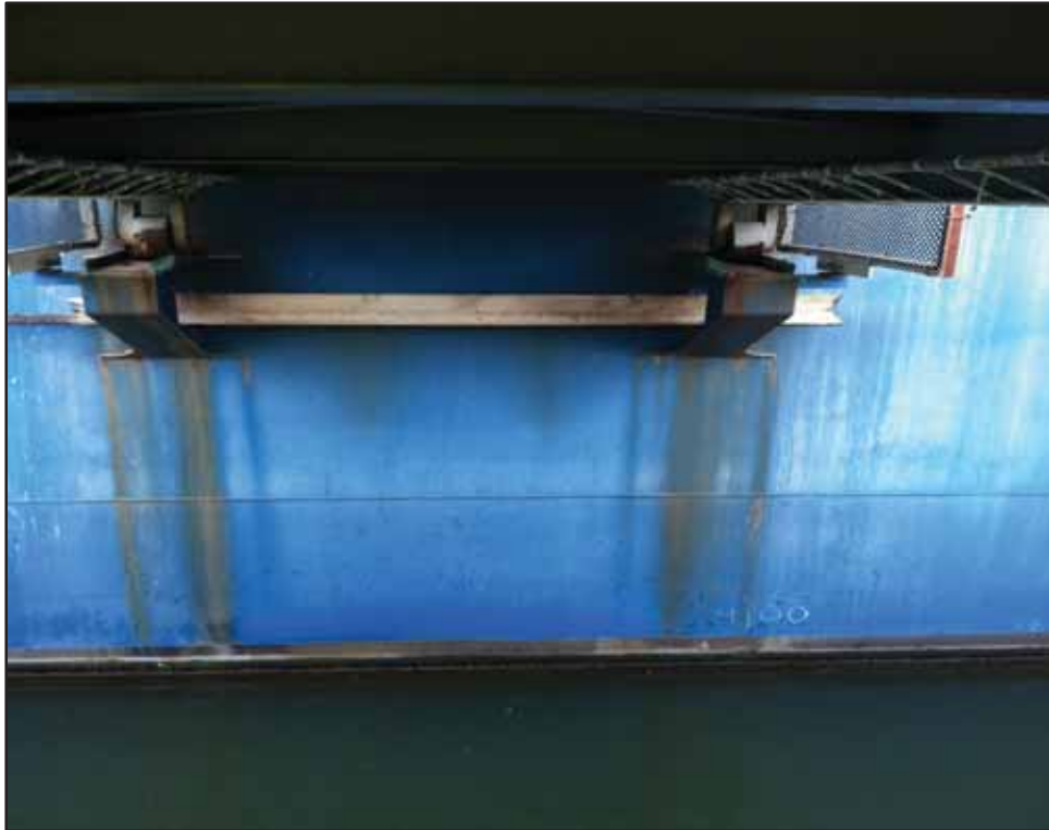
Photo 15-Rollers and underdeck of gangway at Station 7 + 10
