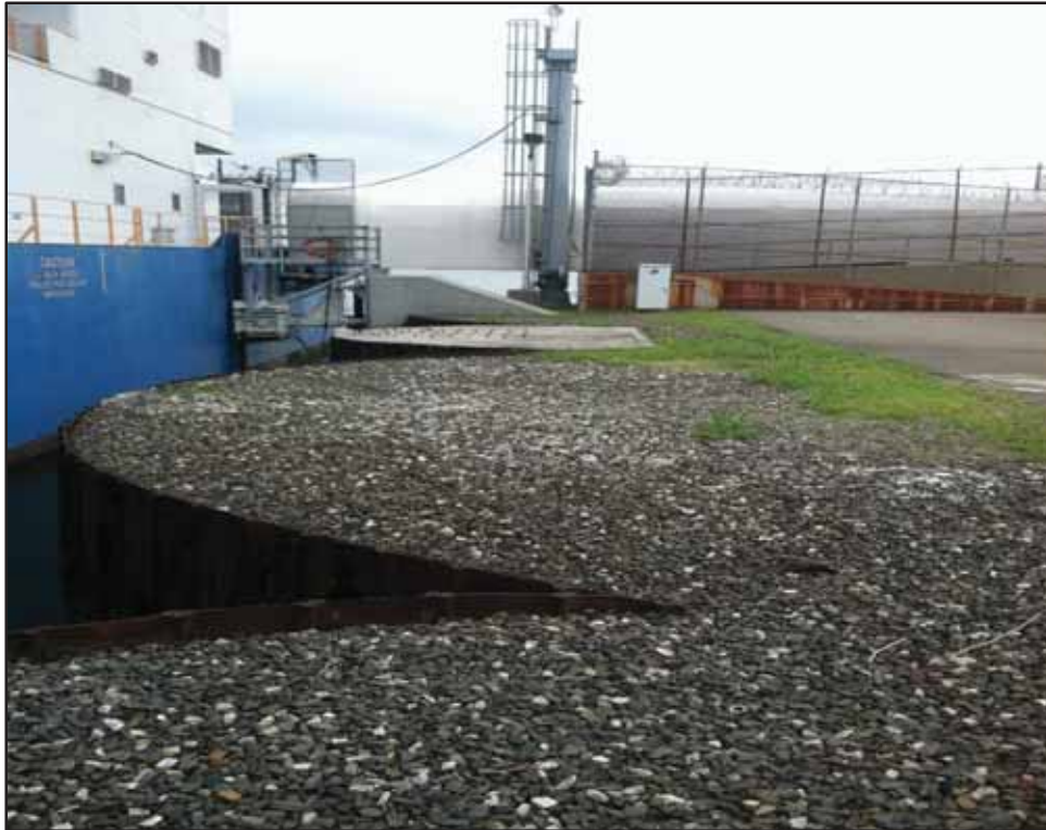
Photo 27-Typical bulkhead on south side at Station 4 + 40 looking west
