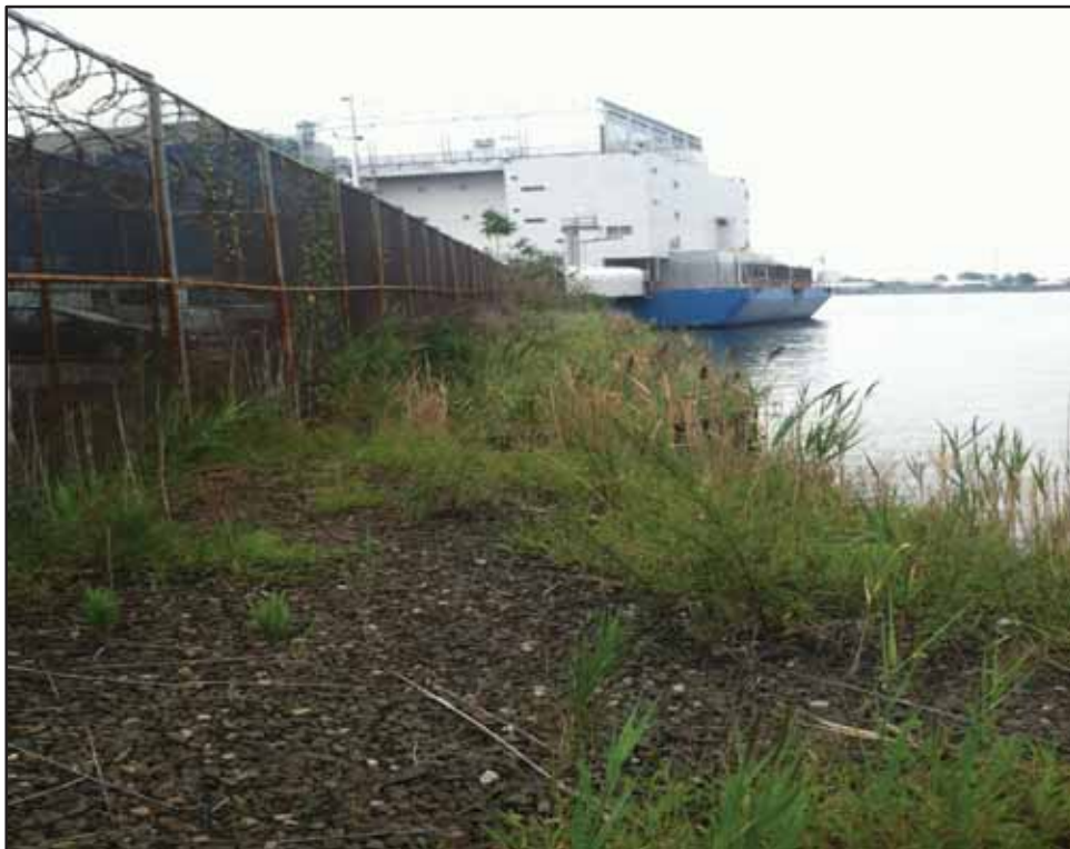
Photo 26-Typical bulkhead on west side at Station 0 + 00 looking south
