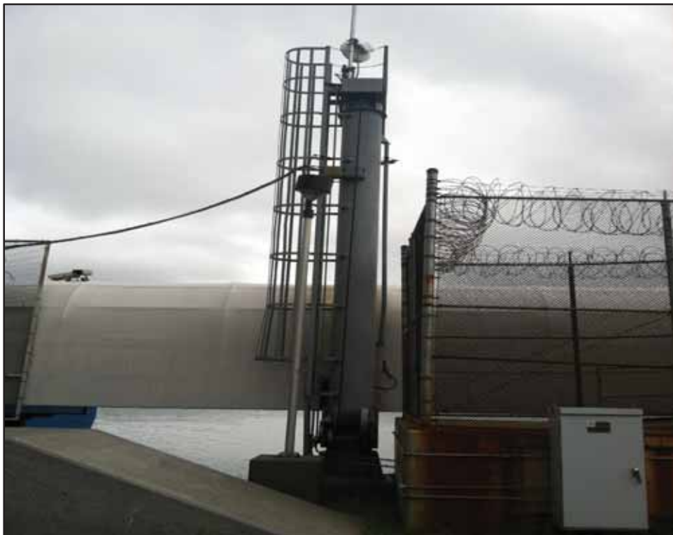
Photo 6-Gangway winch tower at Station 3 + 15
