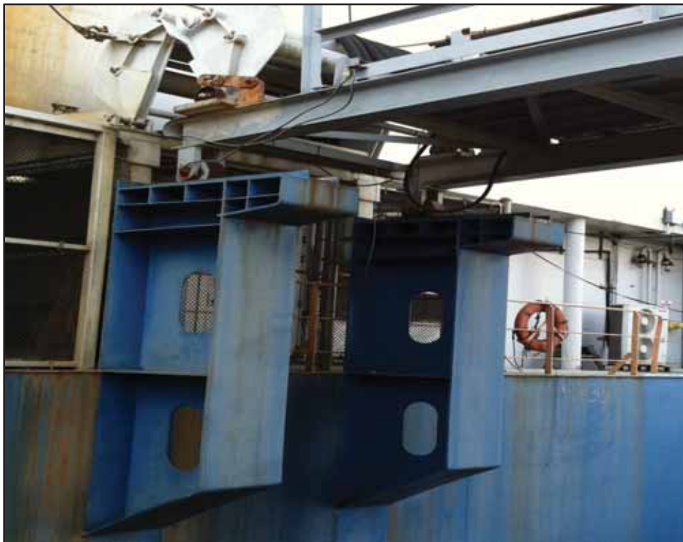
Photo 18-Rollers of utility gangway at Station 7 + 53
