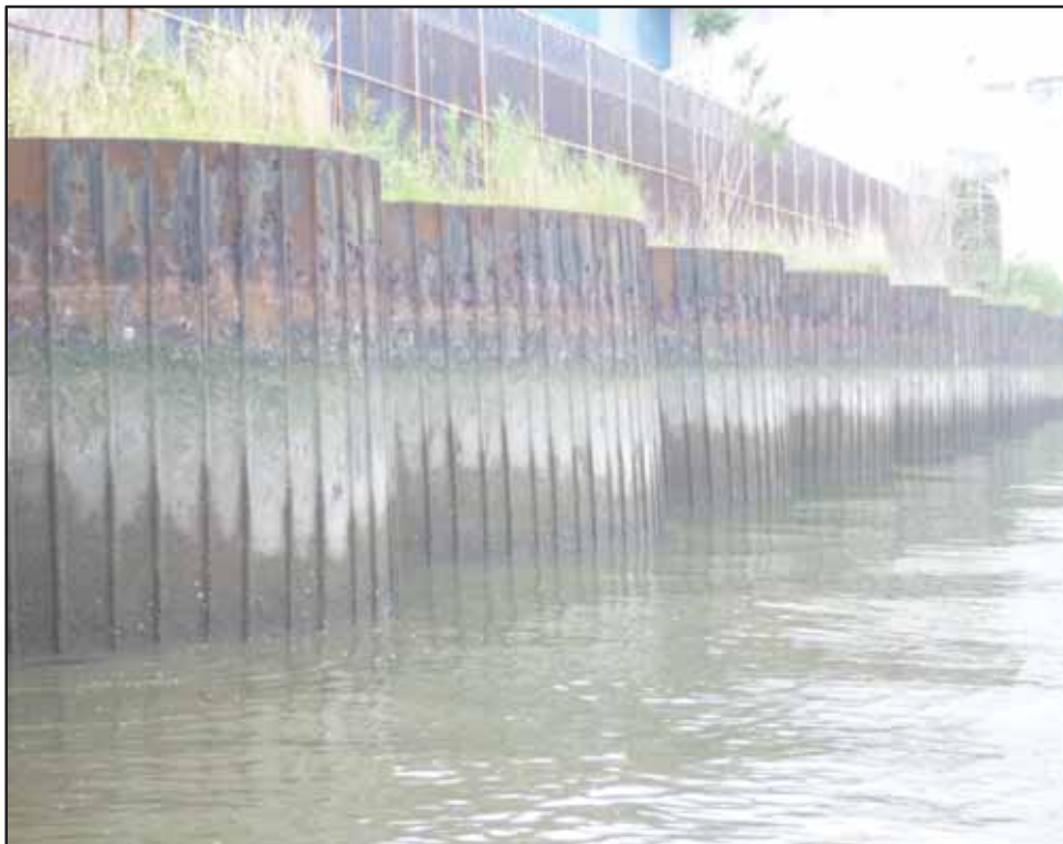
Photo 36-Bulkhead on west side looking south at Station 0 + 00
