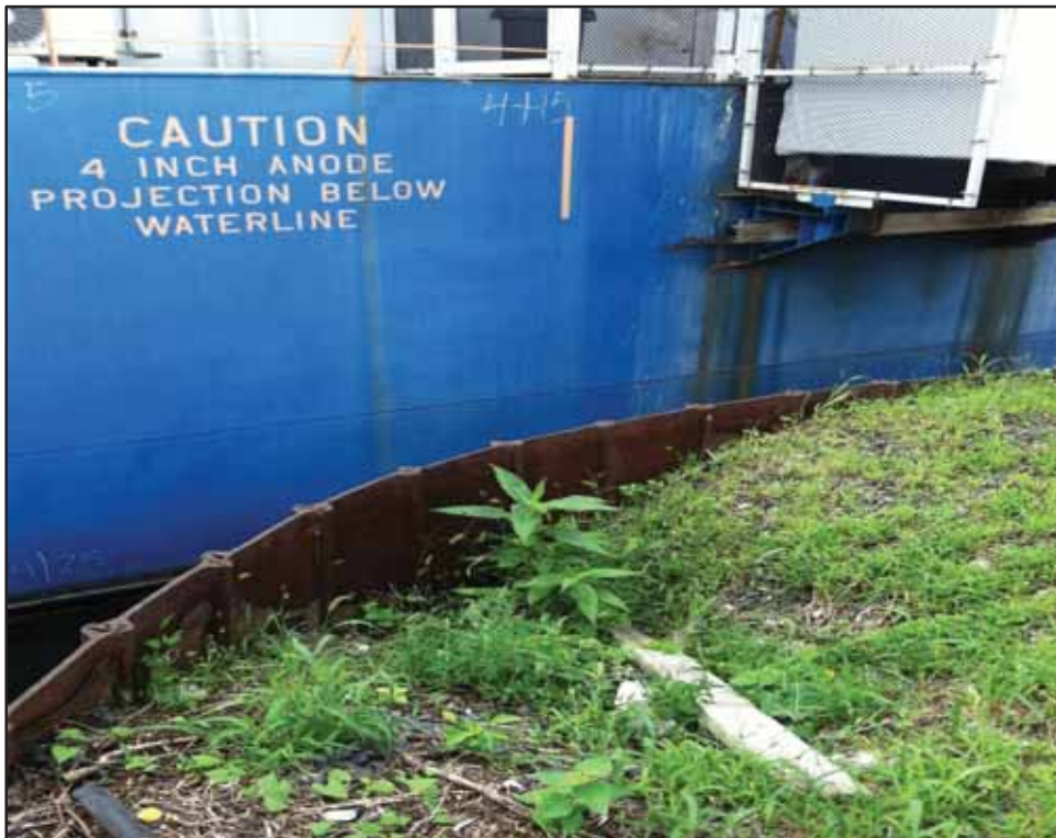
Photo 34-Sinkhole at 7 + 23 9'L x 6.5'W x 2.5'D
