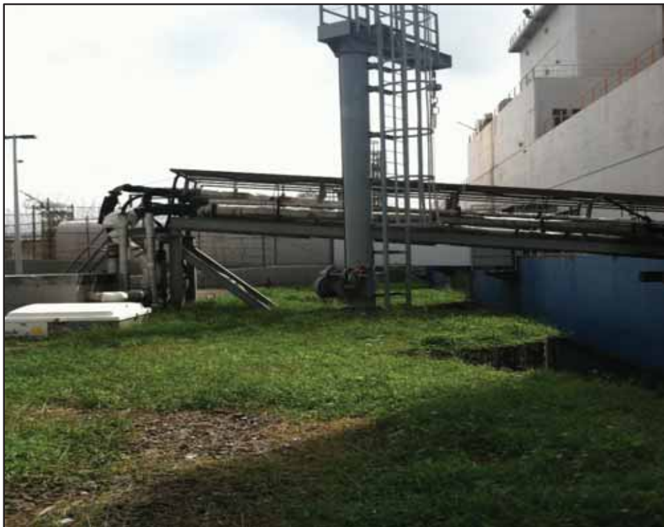
Photo 12-Utility gangway at Station 6 + 71
