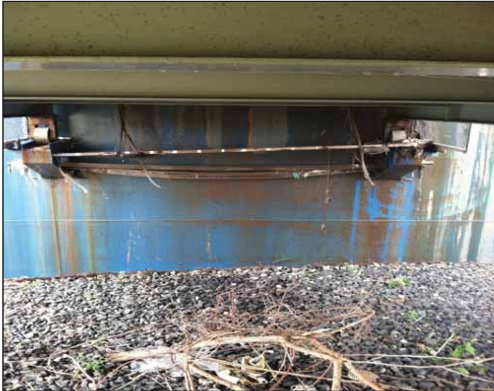
Photo 21-Underdeck and rollers of maintenance gangway at Station 7 + 76
