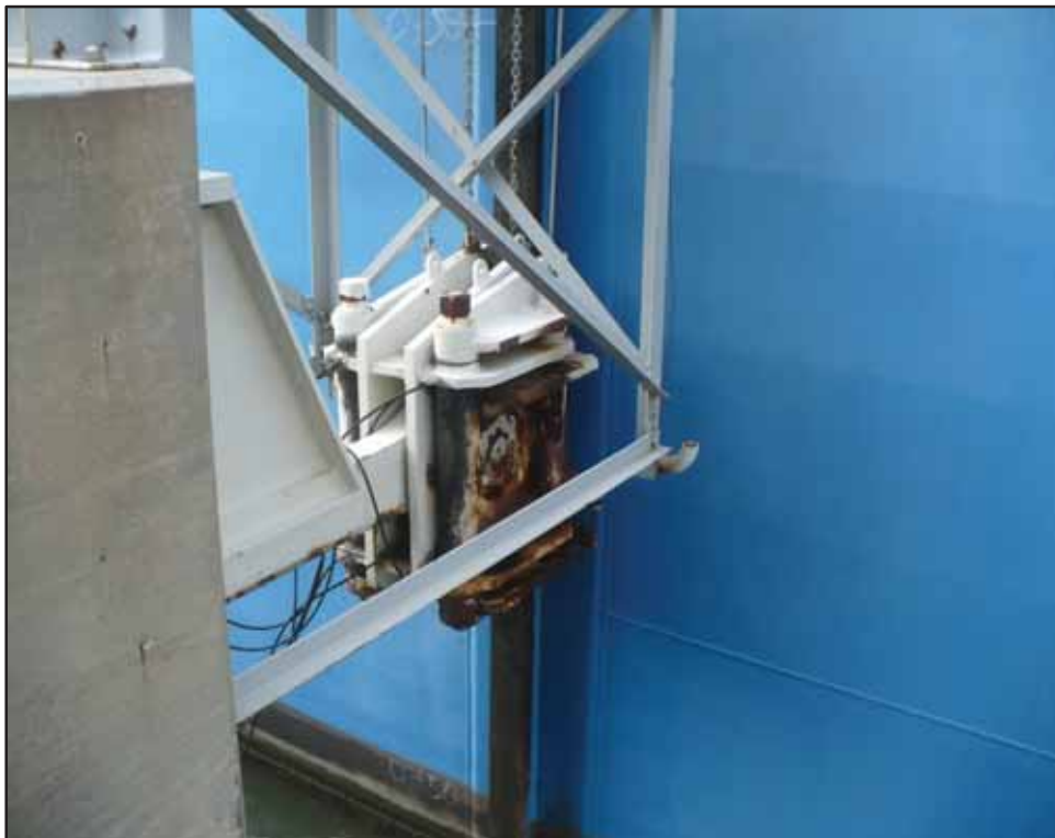
Photo 8-Single mooring connection at Station 3 + 22 looking east
