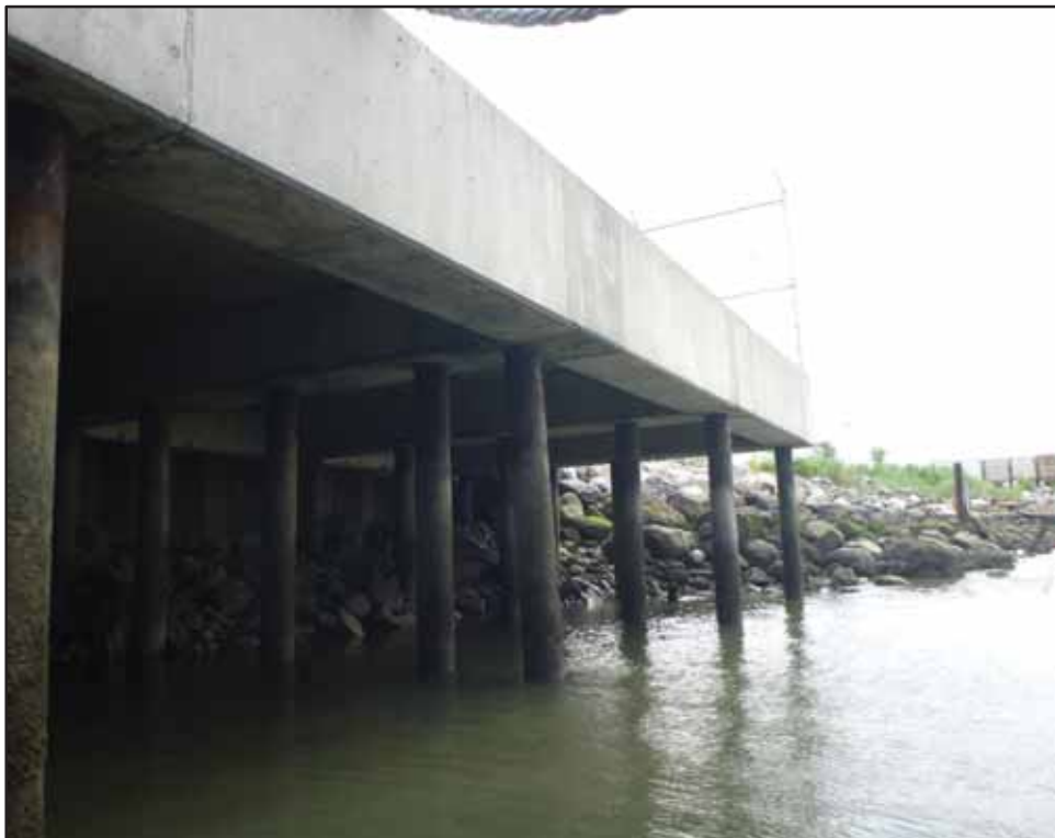
Photo 24-Pile supported platform looking east
