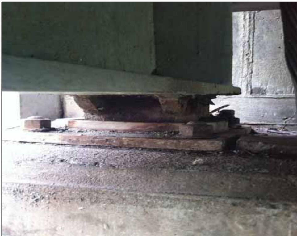
Photo 20-Bearing plate and connection of maintenance gangway at Station 7 + 76
