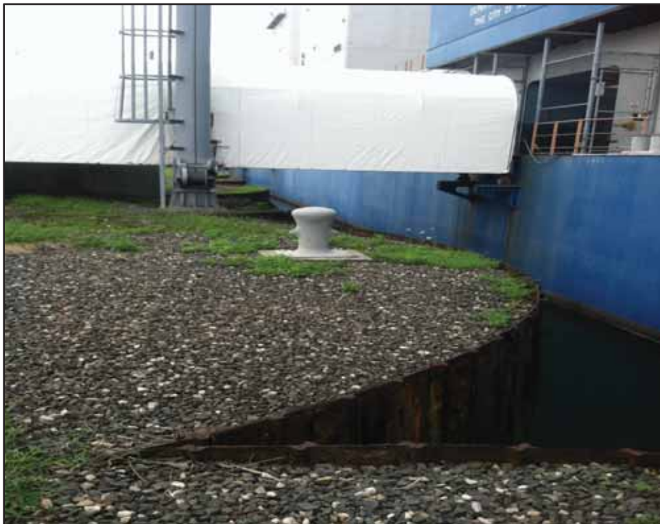
Photo 28-Typical bulkhead on south side at Station 4 + 40 looking east
