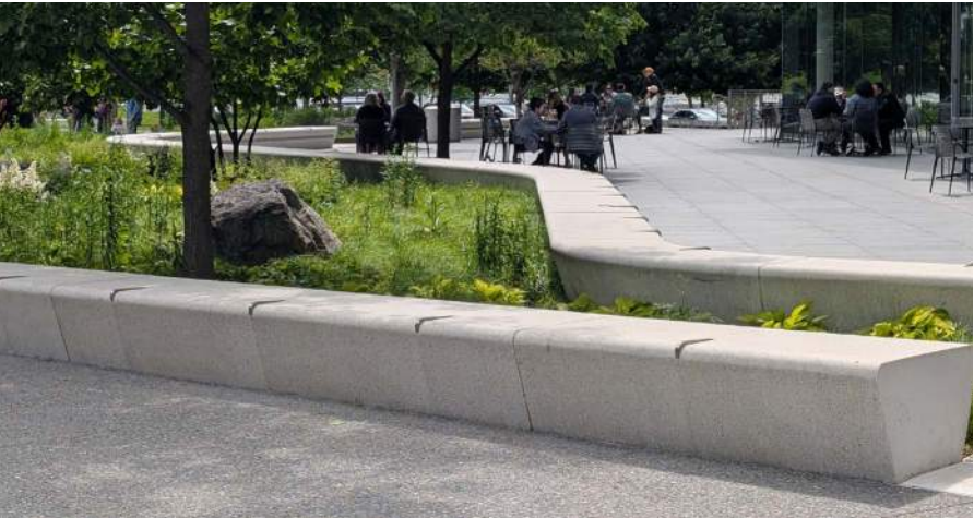
Precast concrete seating wall Cornell Tech Campus, NY
