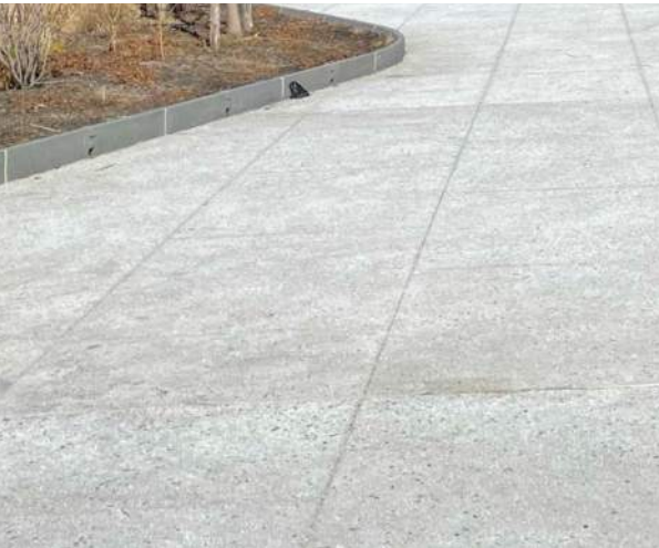
Cast-in-place concrete (Greenpoint Landing, Brooklyn)
