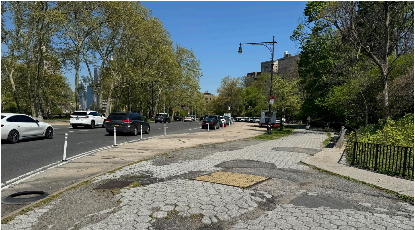
8 - Asphalt hex pavers comprise much of the sidewalk around Grand Army Plaza. Many of these areas are in disrepair
