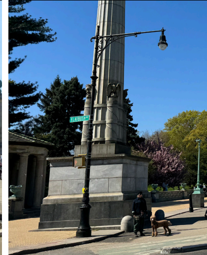
Type M Lightpole (Teardrop Luminaire), 27'-7"
