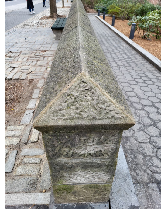
End treatment by CPC on new entrance at E 64 th Street
