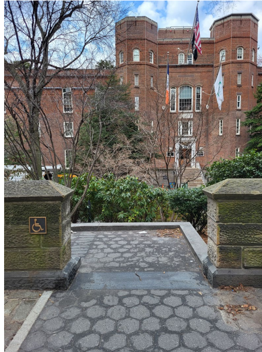
New ADA wall entrance E 64 th Street and Fifth Avenue
