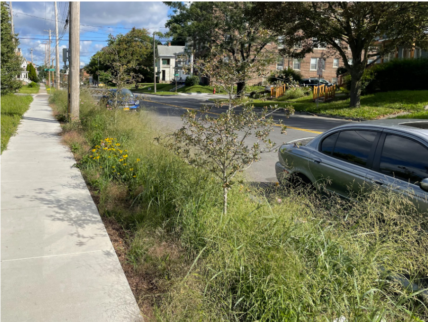
Underground infiltration trench in a grassed and vegetated area, one year after installation, showing a variety of thriving plants
