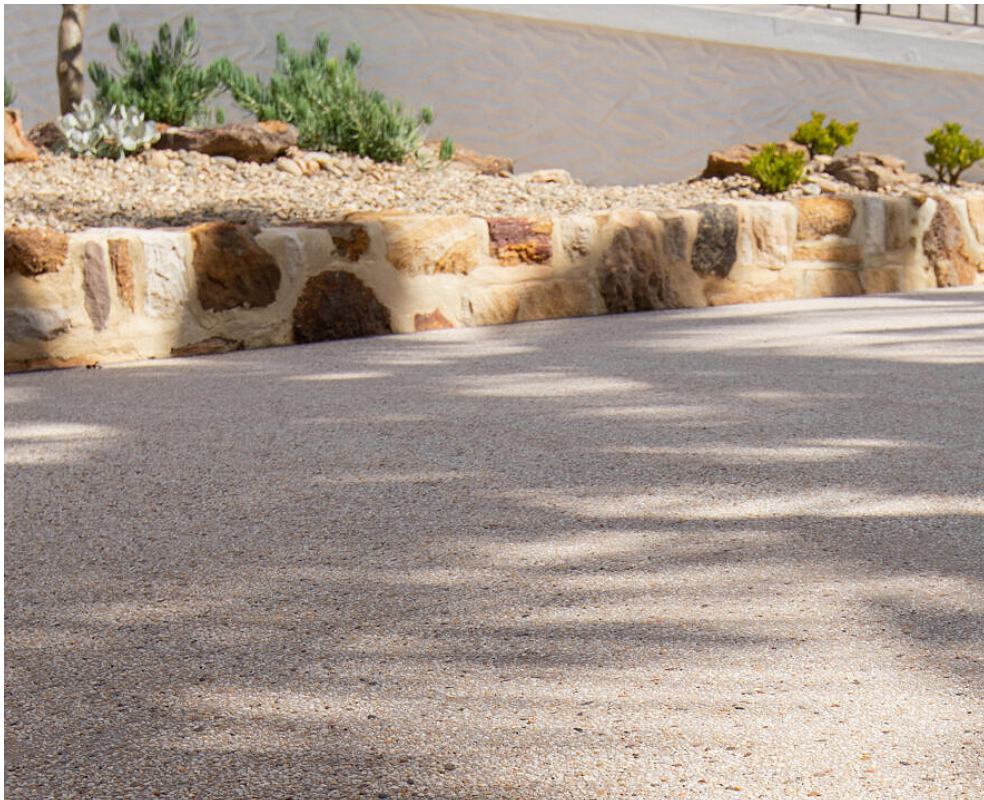
Concrete with Exposed Aggregate - Plazas
