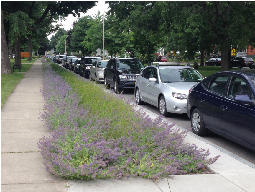
Underground infiltration trench with 2-3 year growth after installation
