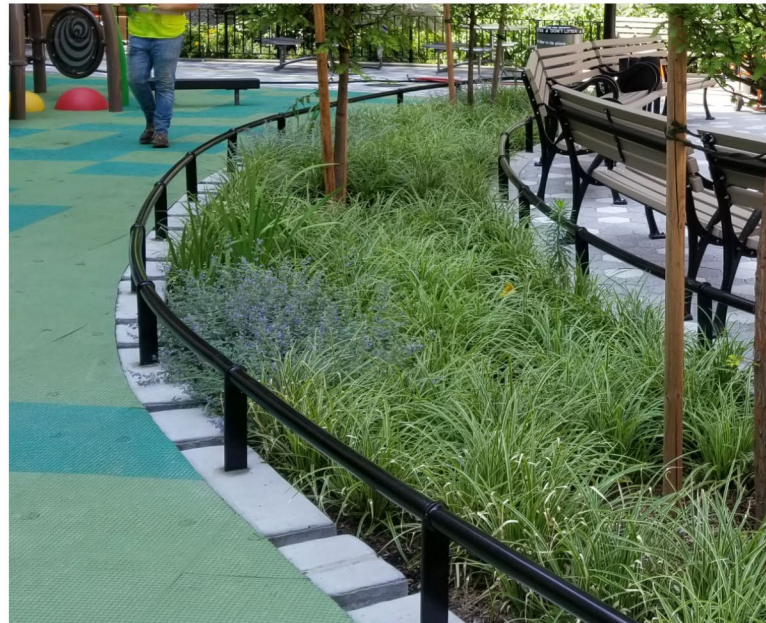
Low Plant Rail (1' - 4" ht.) on Flush Curb
