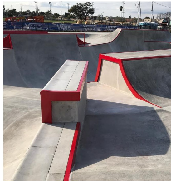
Protective Edging for Transition Elements Steel Coping, Pool Coping and C-Channel (for vertical protection)**
