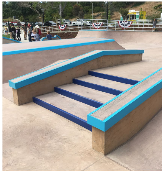
Protective Edging for Street Elements Steel C-Channel**
