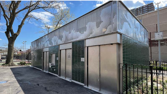
4 Frederick Johnson Park Comfort Station Manhattan Department of Parks & Recreation NYC Parks In-house Design
