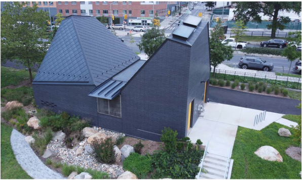
5 Starlight Park Comfort Station and Garage Bronx Department of Design and Construction Department of Parks & Recreation Gray Organschi Architects
